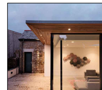
Timber cladding to eaves and end wall
