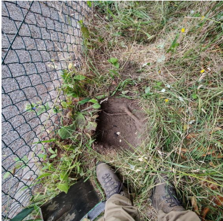
Photograph 12- Trial Pit 4 located adjacent to tennis court and 4m north of trial pit 3. At 100mm in depth, roots of 35mm and 10mm in diameter discovered.
