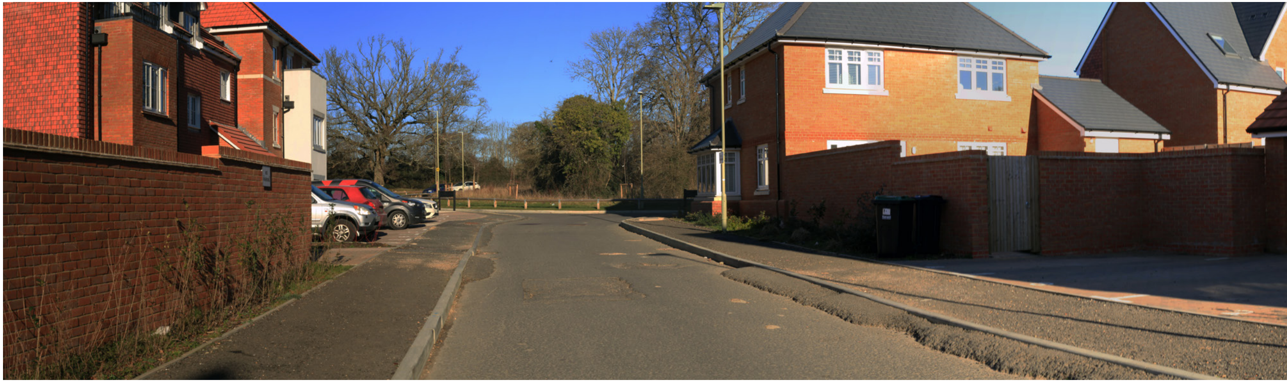
View 9: From Coddington Grove to the south of the Site, looking northwards towards the Site. Mature hedgerow vegetation and buildings in the foreground provide good screening, however there is a view through to part of the Site’s western field and at the end of the street.
