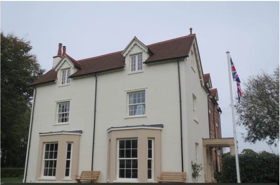
Figure 11: The south-west elevation of Langstone Lodge in 2022
