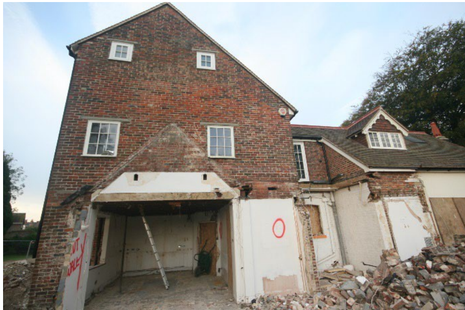
Figure 24: The north-east elevation in October 2023
