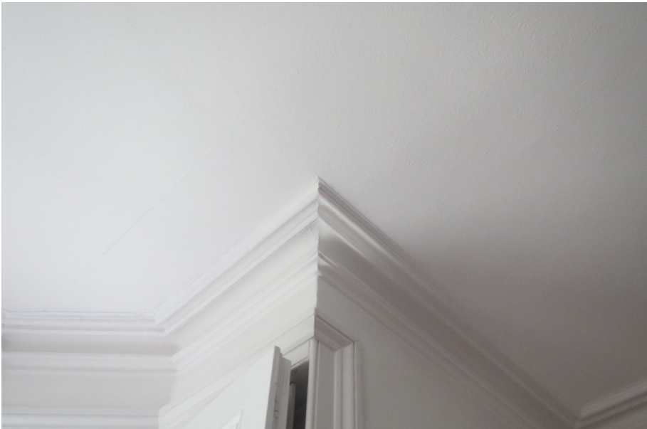
Figure 15: Some of the original plasterwork survives, including the coving in the original range of the building.
