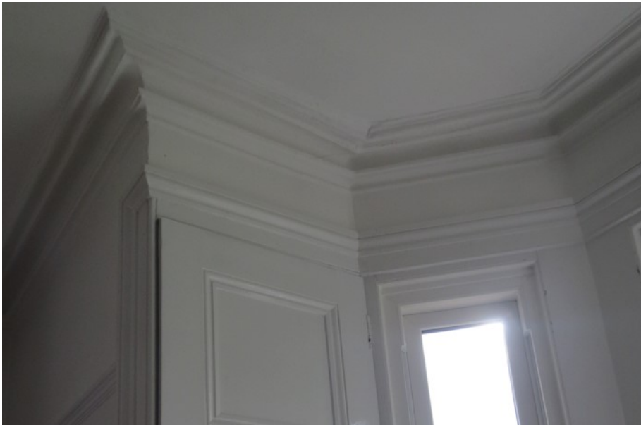
Figure 16: Original coving, window shutters and panelling
