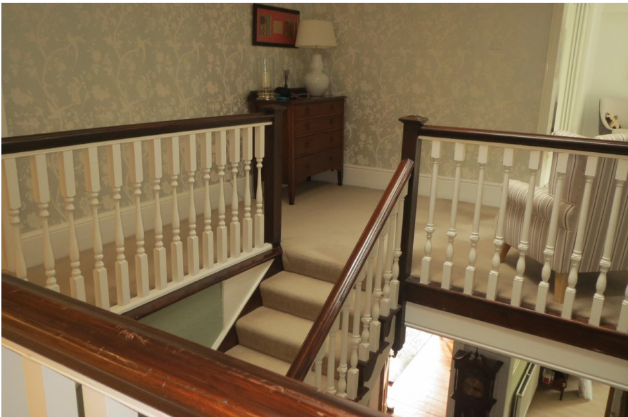
Figure 17: The original staircase
