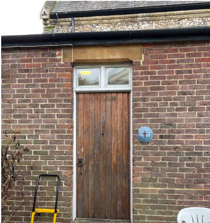
EXISTING DOOR INTO CORRIDOR
