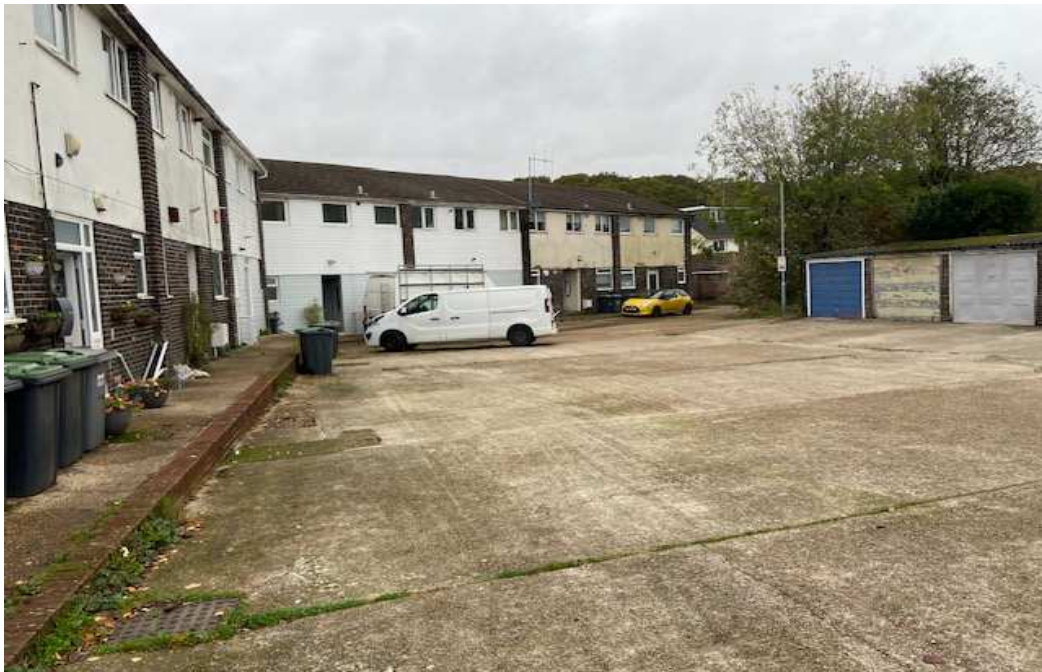
View of the existing commercial area and adjacent garages.
