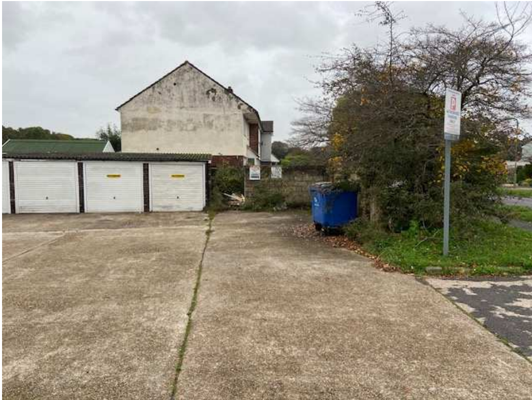
View of the site area looking East
