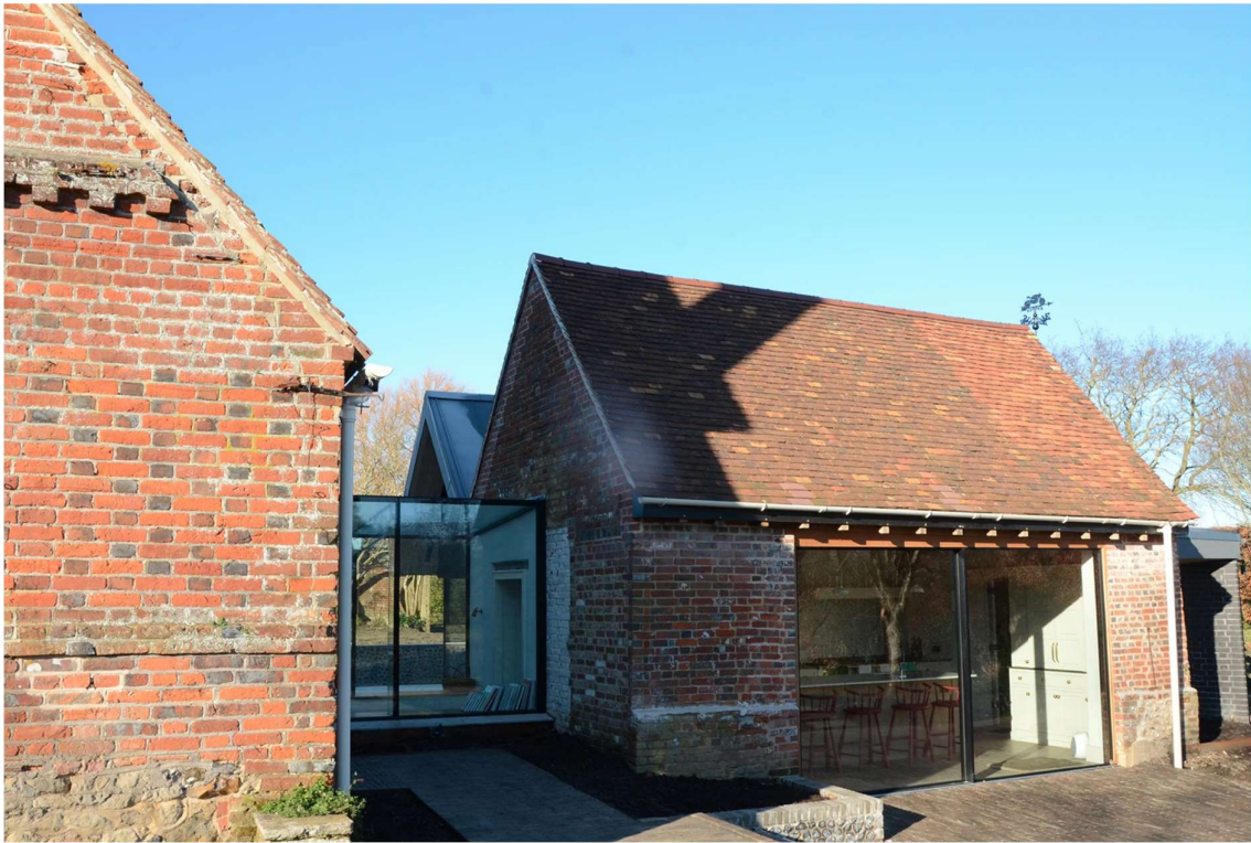
HDS project south of Chichester, Grade II*
