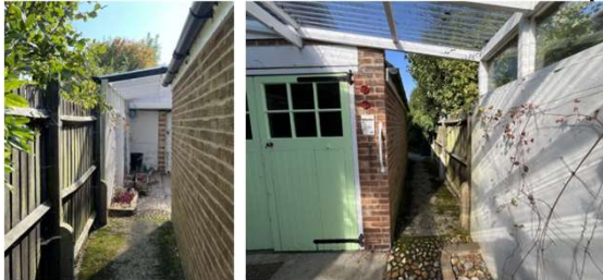
Figure 12 & 13: Shows the existing building at the boundary of the site.
