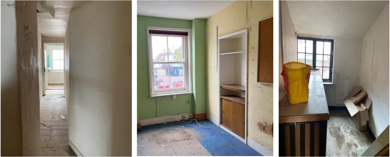
Fig. 07- Left to Right: Existing dwelling hallway to rear existing kitchenette; Existing 'Office B' -window to street view; Existing 'Office B' over ground floor side access looking to rear of property.
