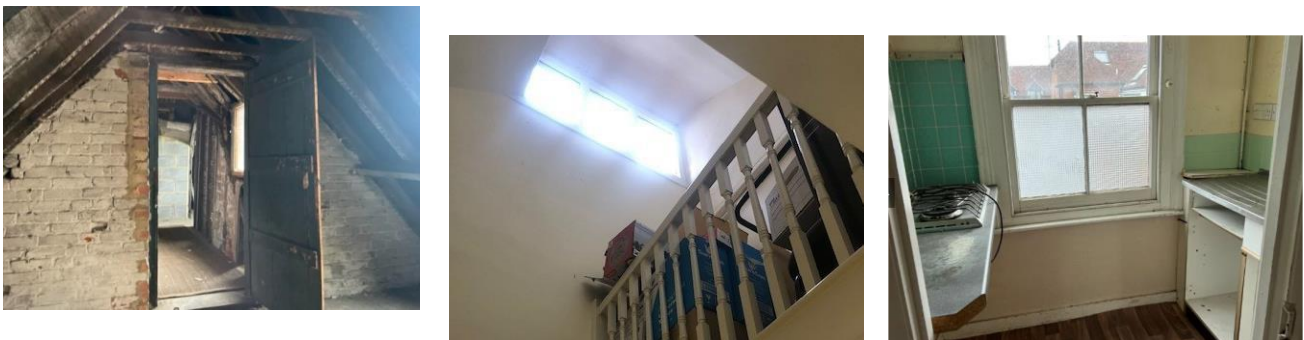
Fig. 08- Left to right: Existing loft space, currently as part of 'Office B' ; Existing Dormer to 'Office A' stairwell- interior view ; Existing dwelling kitchenette
