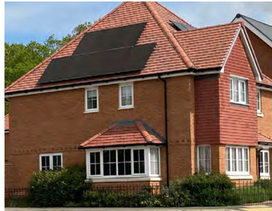
Use of photovoltaics at Catherington Park
