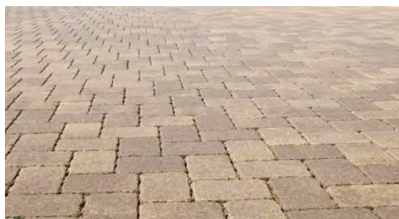
Block Paving - used in courtyards and shared space areas
