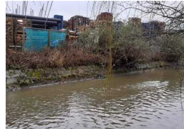
VIEW - 3 (HERMITAGE STREAM)
