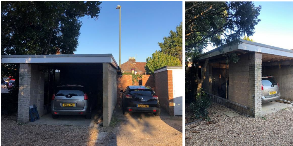
Figures 13 & 14: Garage – (Currently under construction improvements)
