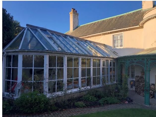
Figure 10: Orangery to the rear of Seafeld House.
