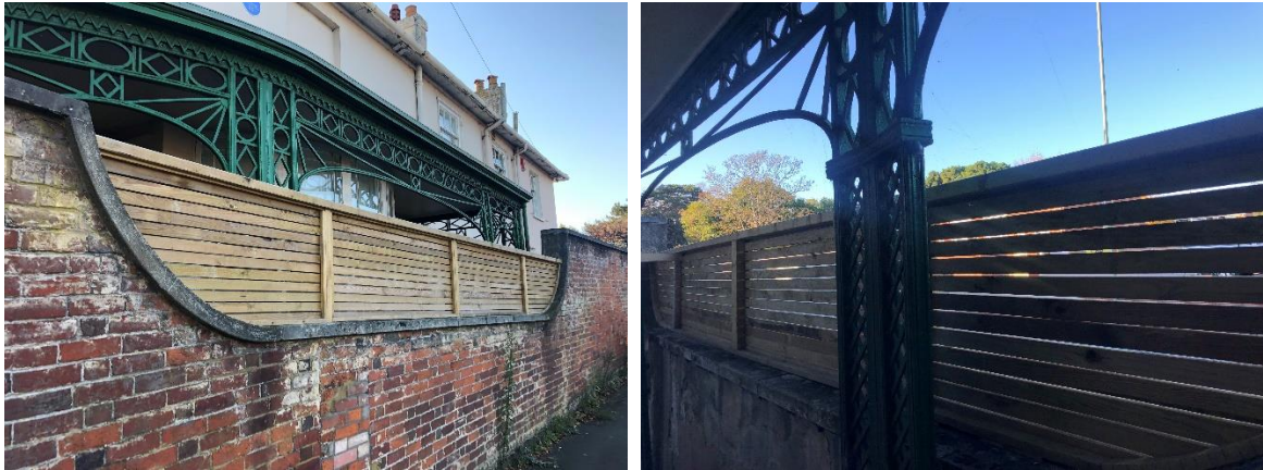
Figures 11 & 12: Fencing to wall on Street Elevation
