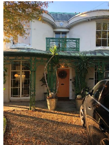
Figure 8: Front Door on East Elevation
