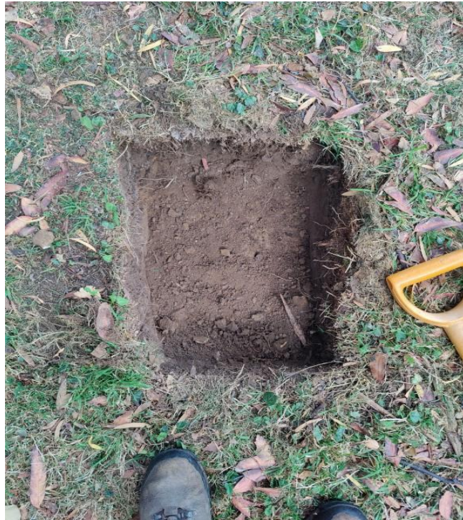
Photograph 3- Trial pit 1: continuation to 100mm, only fibrous roots found.
