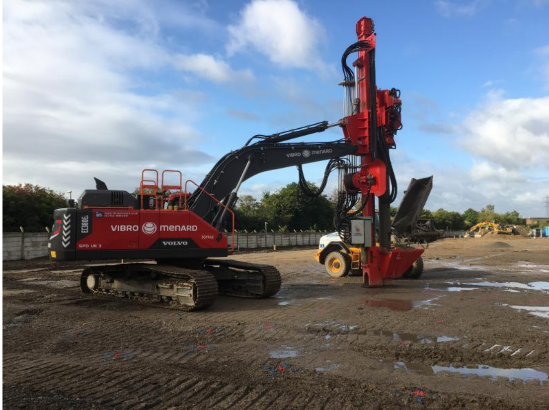
Figure 3 – VSC rig on site
