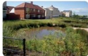
Examples of sustainable drainage pond at Broomwood, Watlingtonville Grainger PLC
