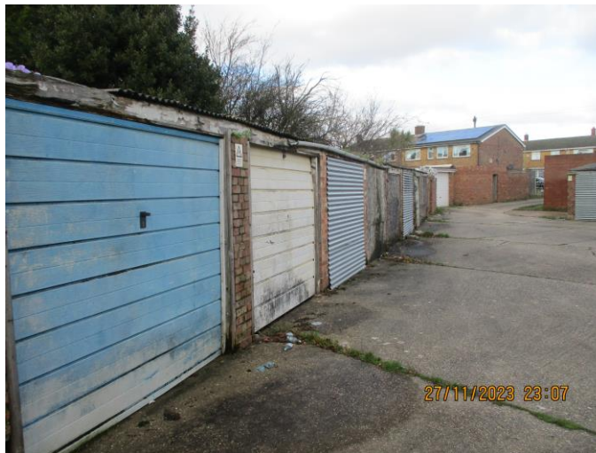
Photo 2: West row of garages (B1).
