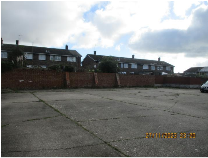
Photo 7: Garage compound (u1b).
