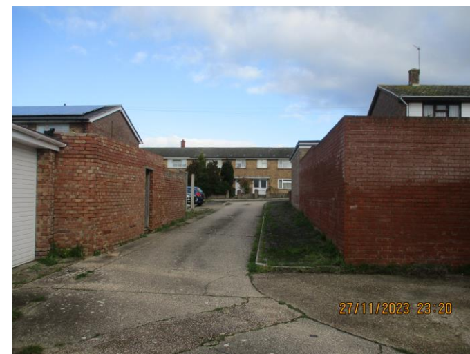
Photo 6: Garage compound driveway.
