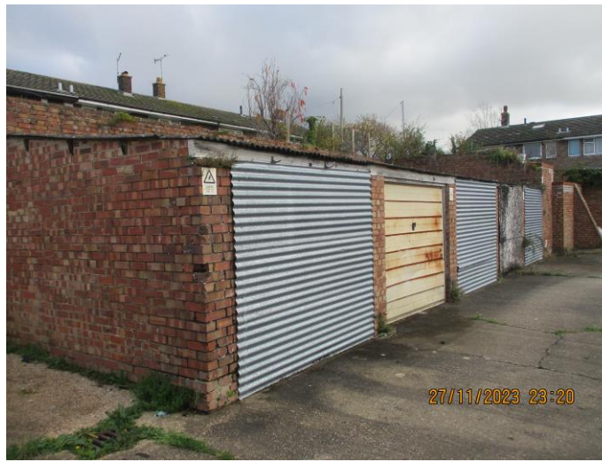
Photo 8: West row of garages (B2).
