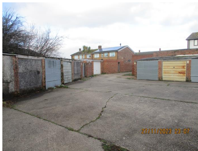
Photo 5: Garage compound (u1b).
