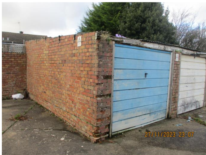
Photo 1: West derelict garages (B1).
