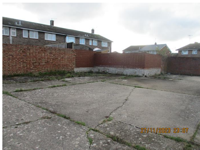
Photo 4: Garage compound (u1b).
