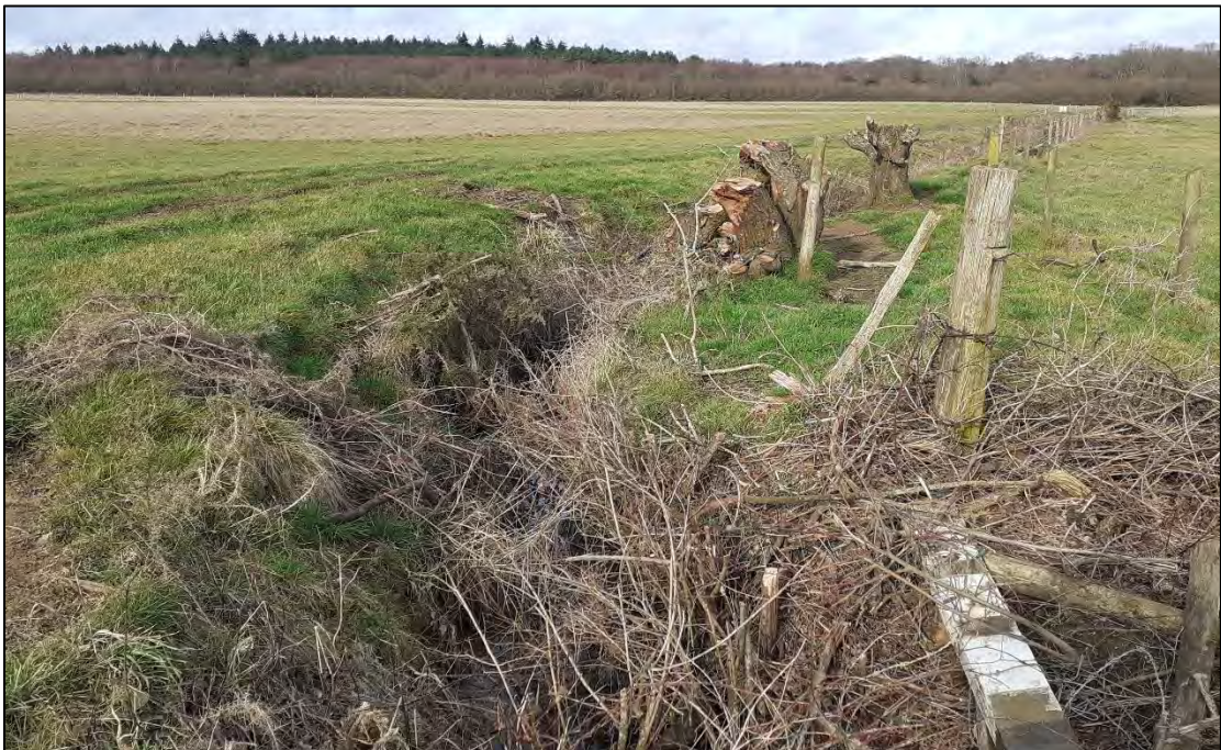
Plate no.8 – Location H, looking north.
