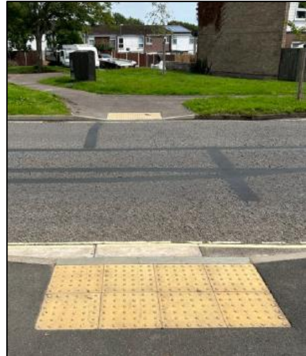
Photograph 13: Crossing Point along Eagle Avenue
