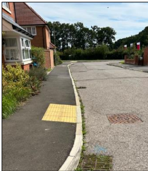
Photograph 8: Footways along Merritt Way
