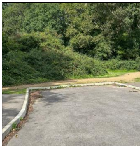
Photograph 2: End of Road at Merritt Way
