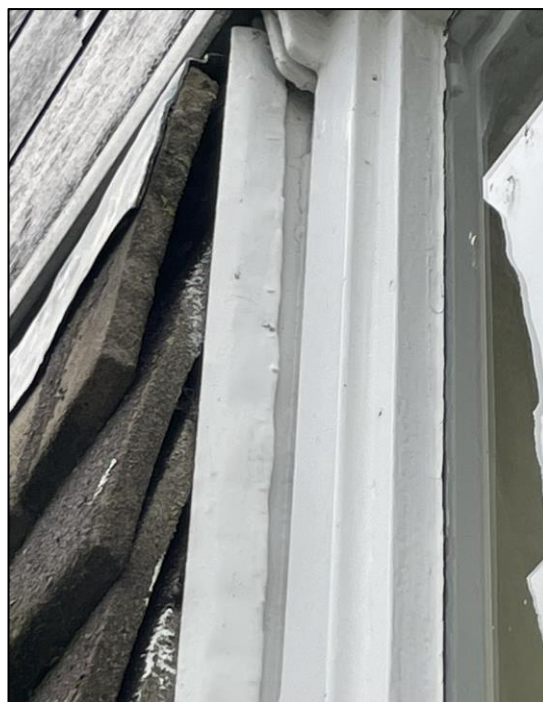
Photos 13 and 14 PRFs C and D – gaps along edges of hanging tiles where they meet the the northeast window corner and window frame. Photo 15 shows the north edge of the window where it meets the corner of the two-storey section; photo 16 shows the south edge of the window, further along the east elevation.
