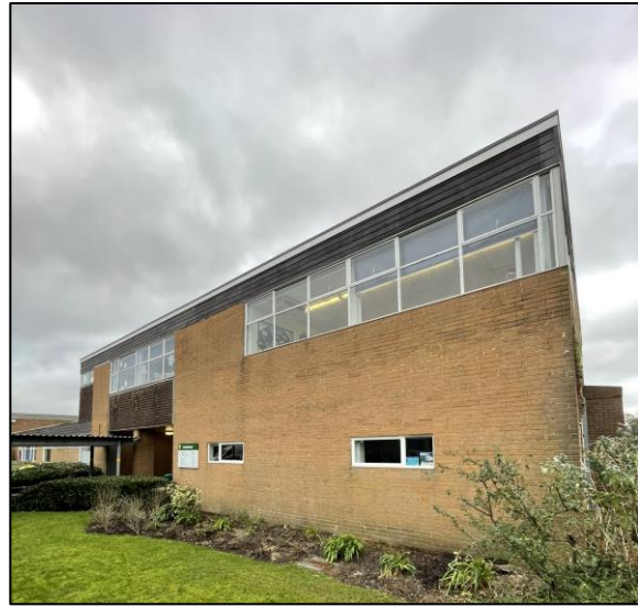
Photo 2 West elevation of two-storey section of Goodwood Block.
