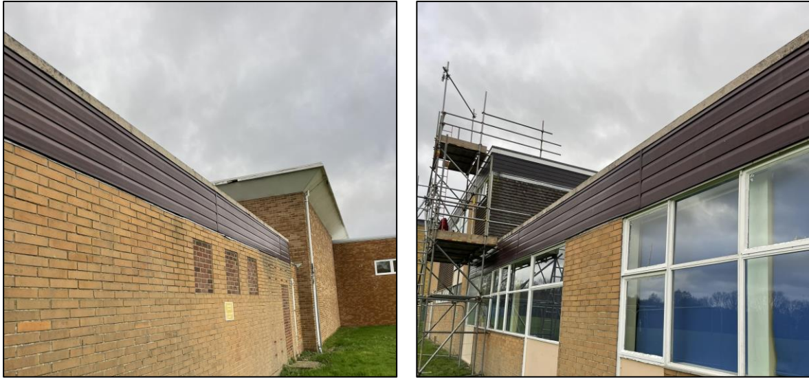
Photos 6 and 7 Views north and south along east elevation of single storey section; timber cladding above windows, typical of that around the building exterior, appears in good condition.
