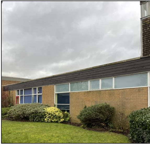
Photo 1 West elevation of single-storey section of Goodwood Block.
