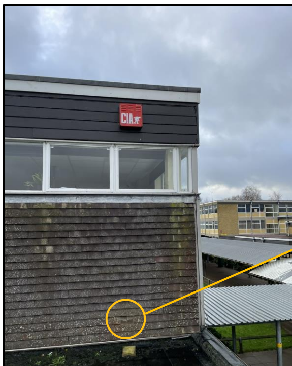
Photos 9 and 10 PRF A - missing tile to southern side of north end of two-storey section.
