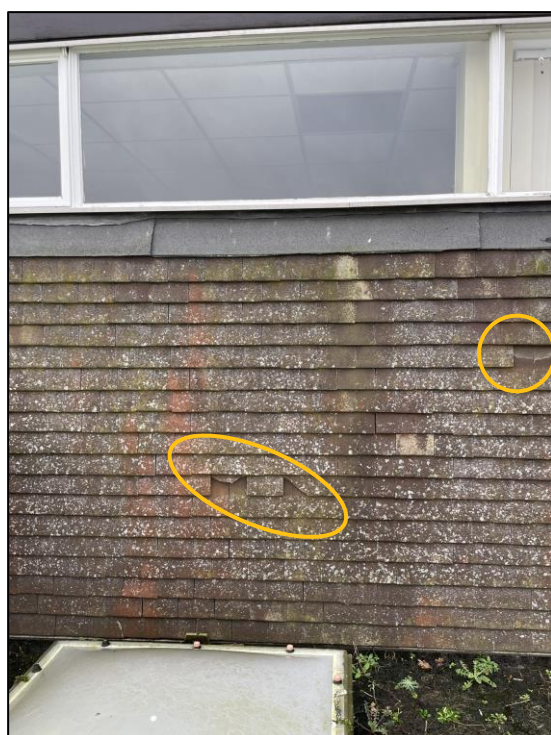
Photos 11 and 12 PRFs B1-B2-B3 – missing and damaged hanging tiles to central area of north end of two-storey section; view into gap created by missing tile.
