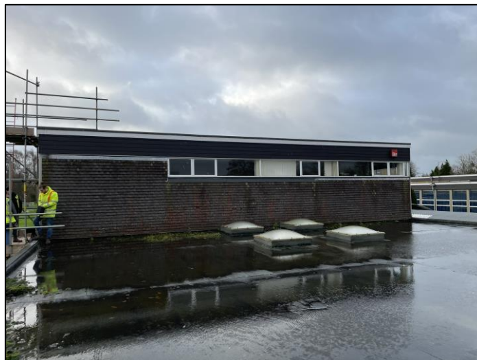
Photo 5 North elevation of two-storey section – viewed from roof of single-storey section.
