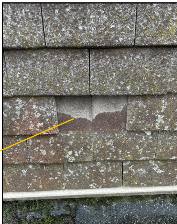
Photos 9 and 10 PRF A - missing tile to southern side of north end of two-storey section.
