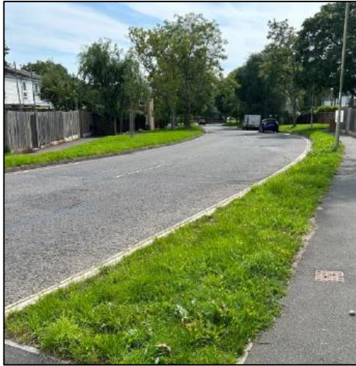
Photograph 12: Footways Along Eagle Avenue
