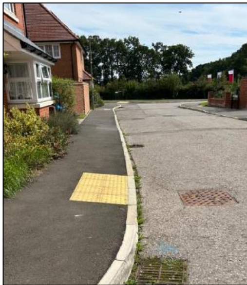
Photograph 8: Footways along Merritt Way
