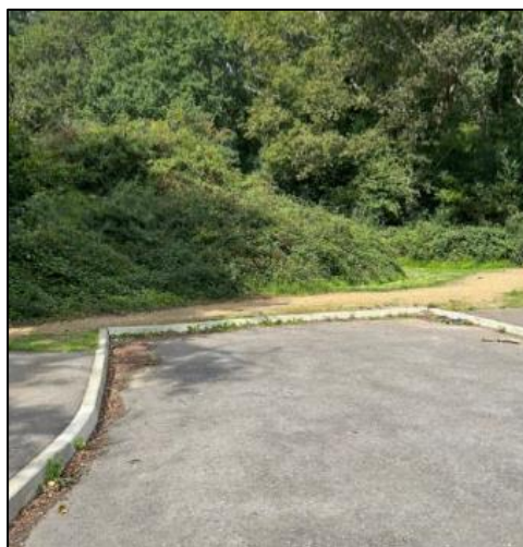
Photograph 2: End of Road at Merritt Way
