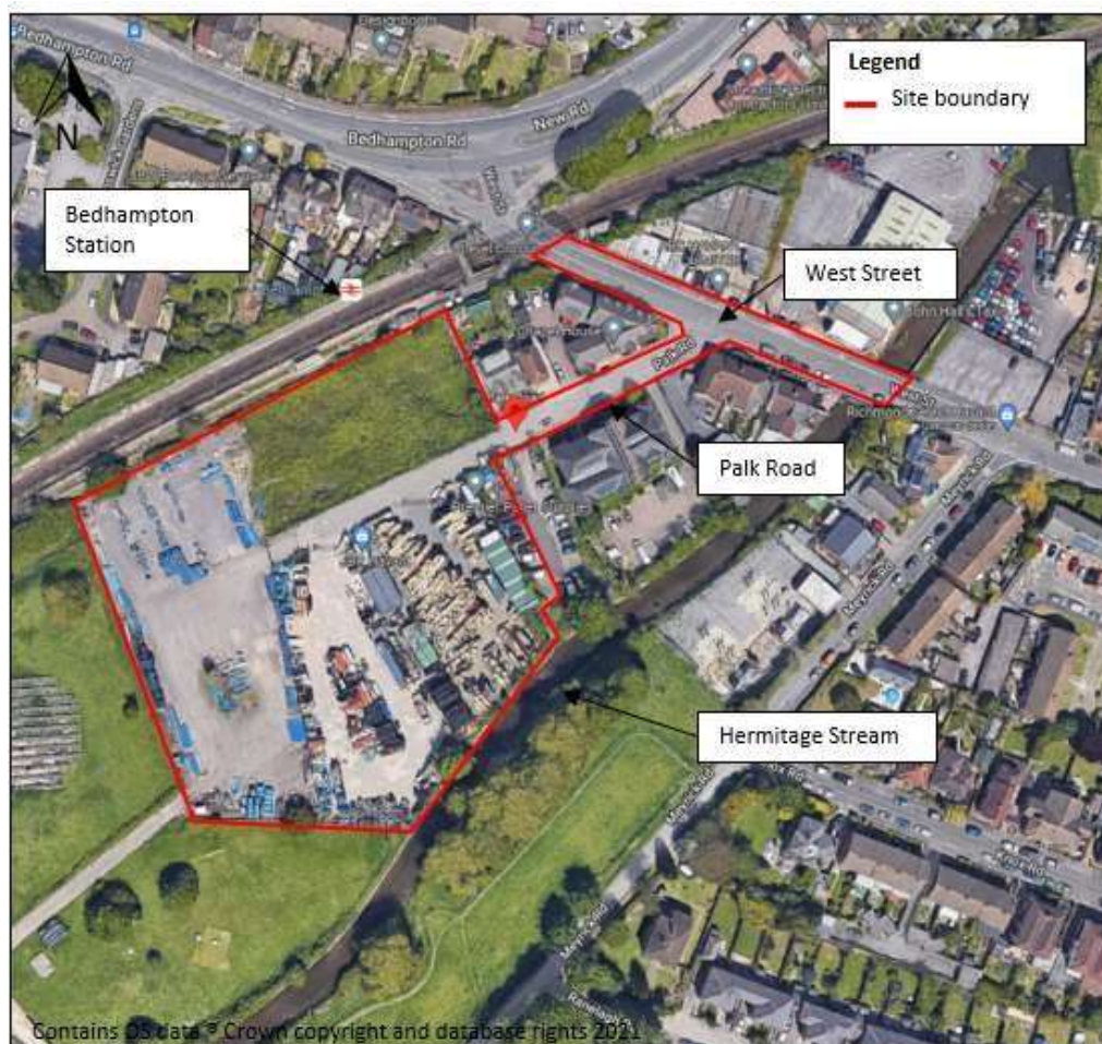
Figure 2-2: Aerial View of the Existing Site
