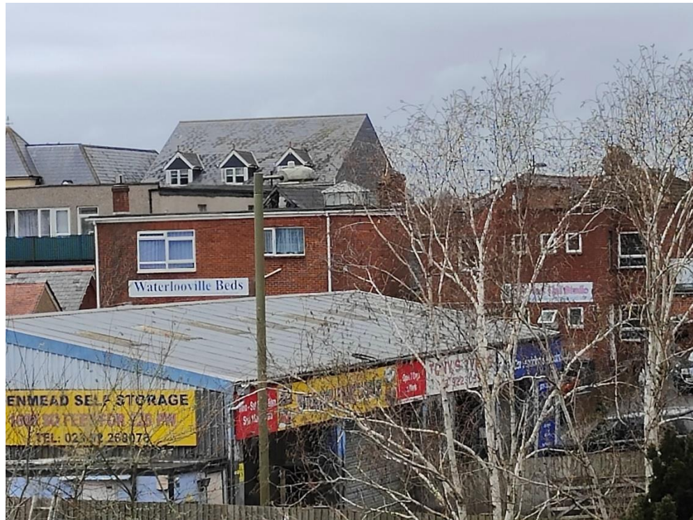
Photograph 1: View of current building from 17 Wellesley Close.
