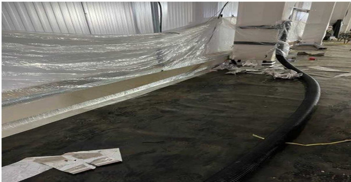
RTEC4 Gas membrane (Black) GRSAM (White) perimeter edge
