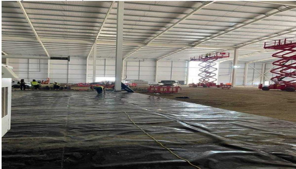
RTEC4 gas membrane (Black)
