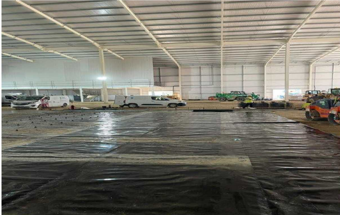
RTEC4 Gas membrane (Black)
