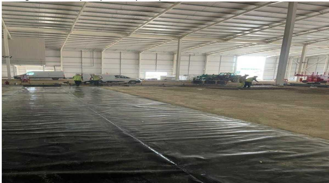
RTEC4 gas membrane (Black) GRSAM (White)
