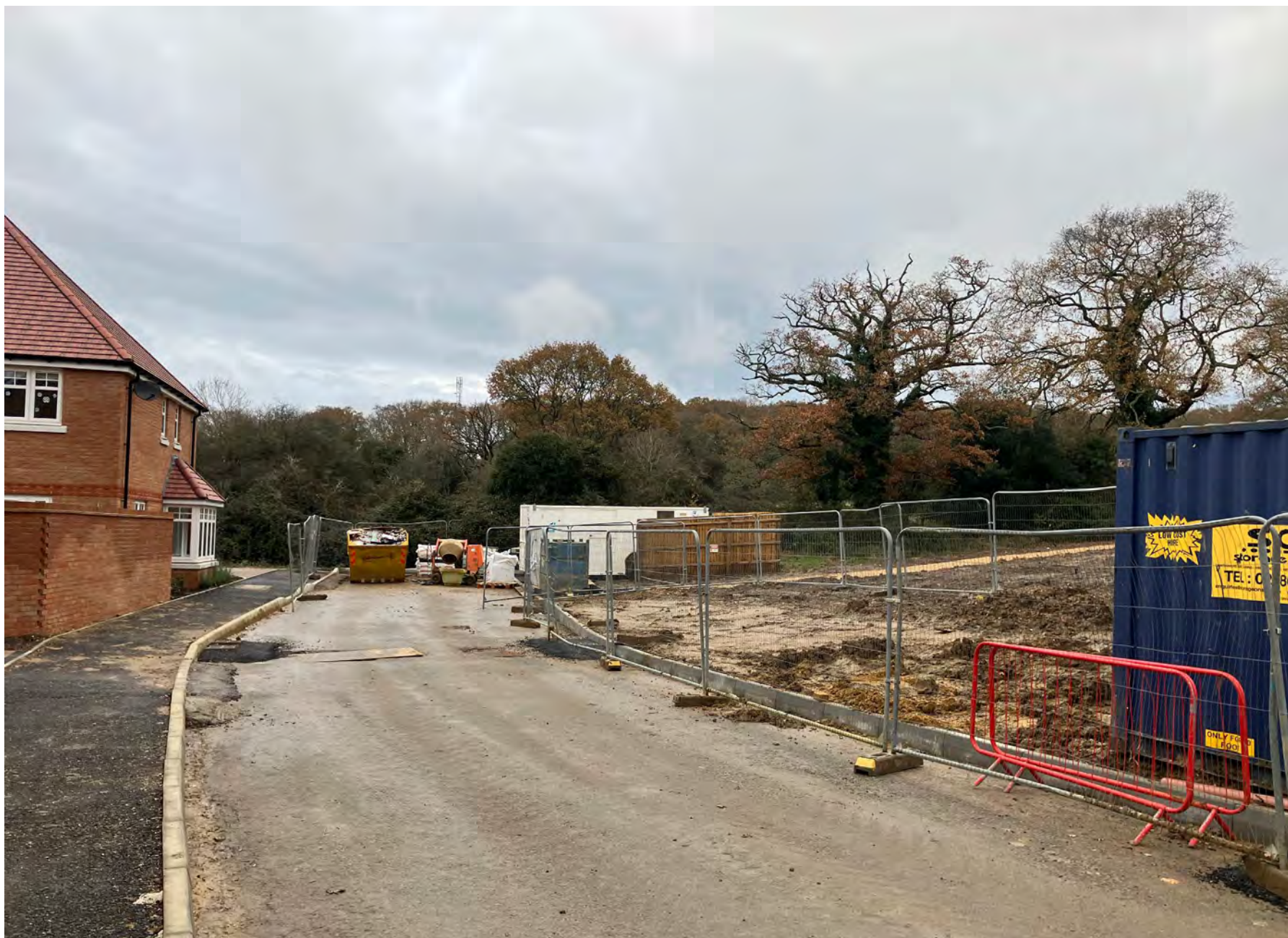
Catherington Park under construction and view towards southern site entrance.
