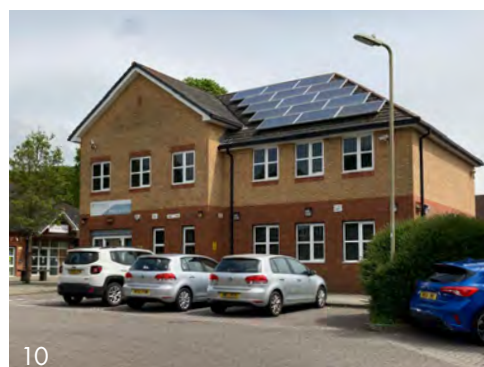
10 The Acorn Community Centre and Wecock Farm Area Housing Office.
