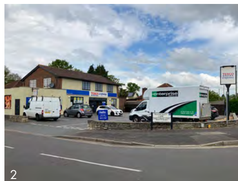
2 Woodcroft Ln and Lovedean Ln local shop.
