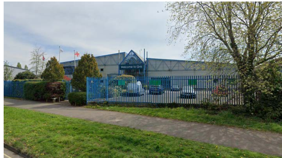
01 View of the pedestrian entrance on New Lane and the main entrance.
