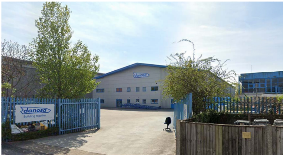
05 Danosa, Stanbridge Road, Havant
