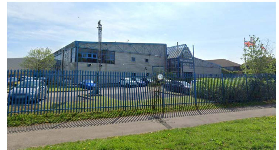
02 View from the post box in New Lane to the main entrance of the Building
