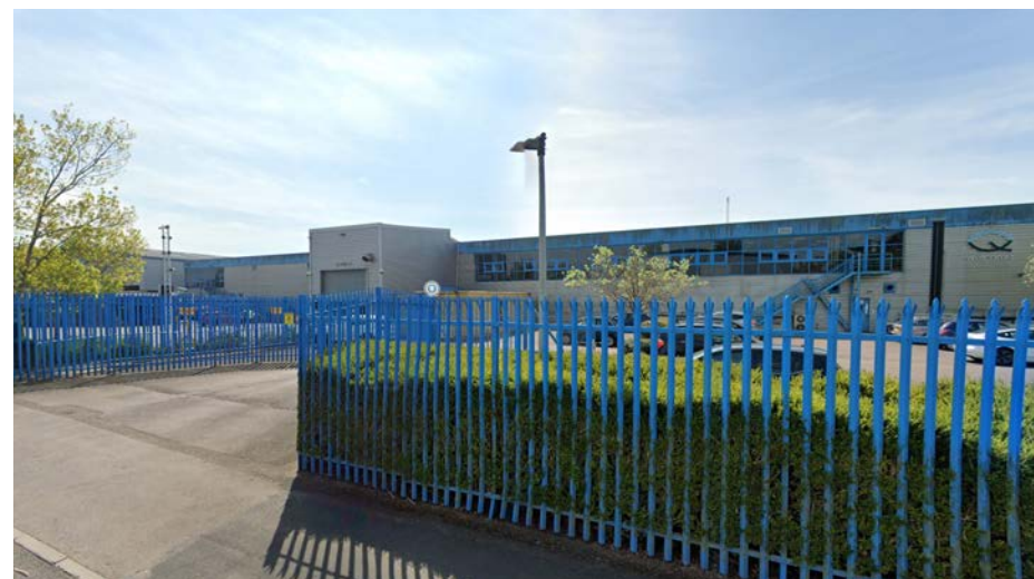
03 View of secondary entrance to the existing building from Stanbridge Road
