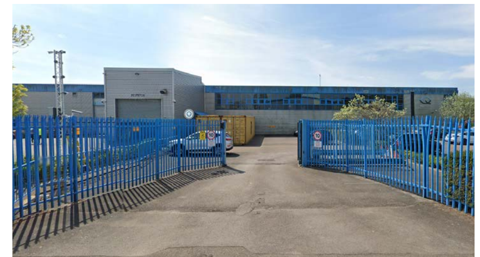
04 View of existing vehicle access from Stanbridge Road.
