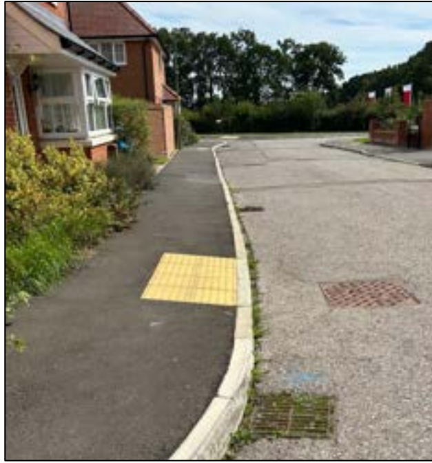
Photograph 16: Tactile Paving along the Eastern Footway of Merritt Way
