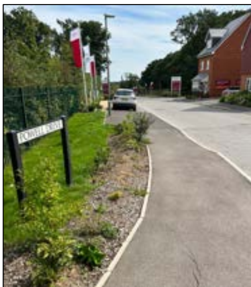
Photograph 6: Footway to the North of Powell Drive
