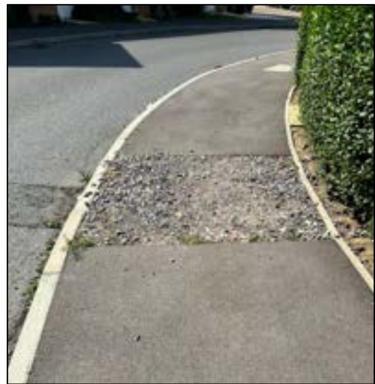
Photograph 19: Existing Conditions along Merritt Way
