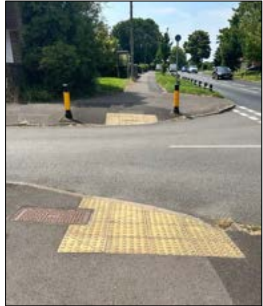
Photograph 76: Crossing Point at Junction along Shared Footway/Cycleway on the Eastern side of Milton Road
