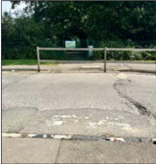
Photograph 10: Existing Road Conditions along Powell Drive
