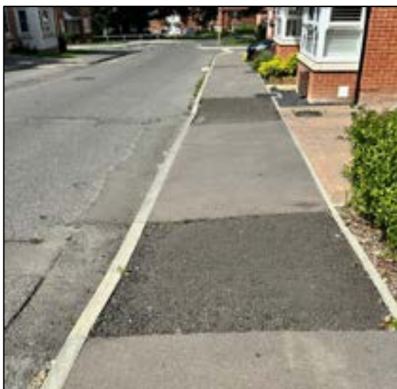
Photograph 20: Existing Conditions along Merritt Way
