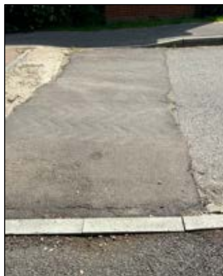
Photograph 21: Dropped Kerbs across Gardiner Walk
