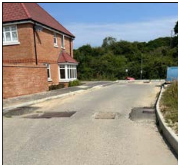
Photograph 25: Existing Conditions along Wilkes Way
