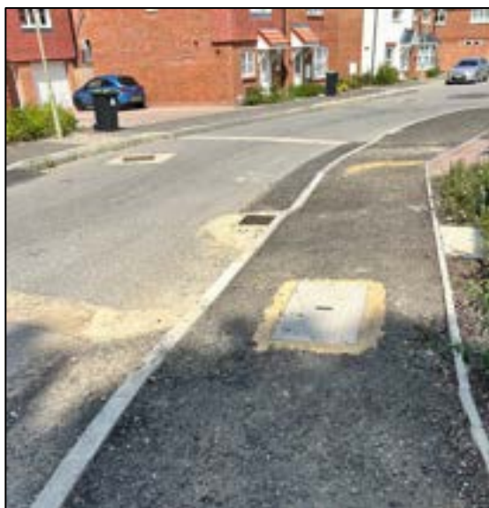
Photograph 24: Existing Conditions along Wilkes Way
