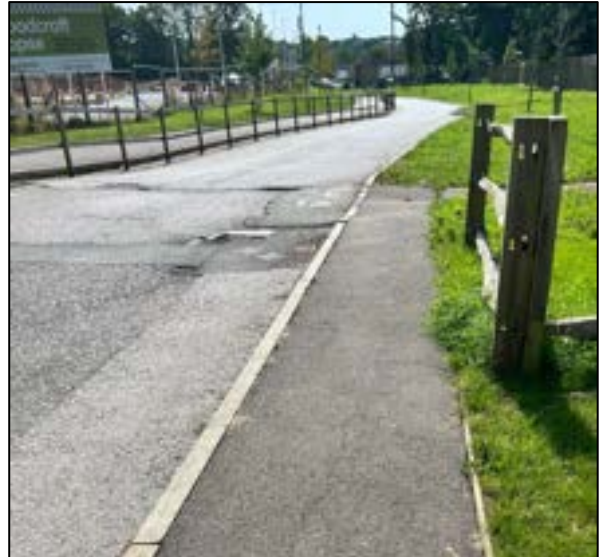
Photograph 11: Existing Road Conditions along Powell Drive
