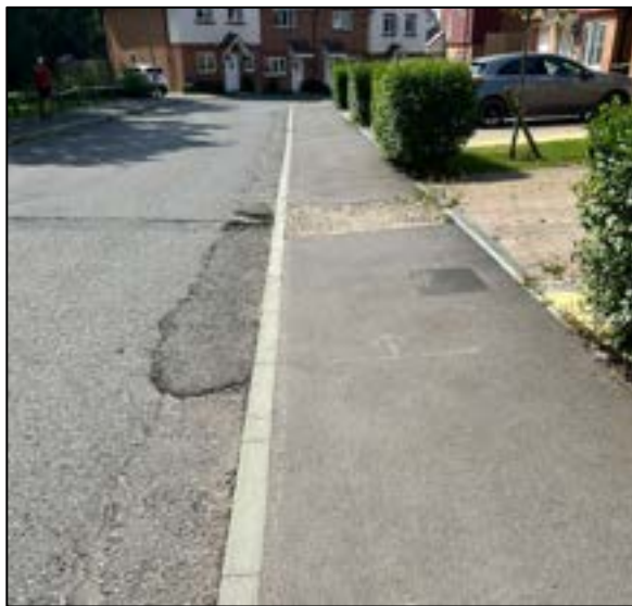
Photograph 18: Existing Conditions along Merritt Way
