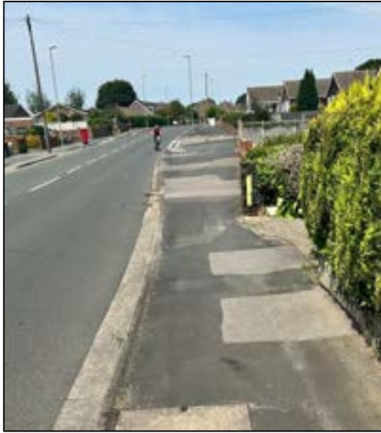
Photograph 66: Hart Plain Avenue South of One Stop
