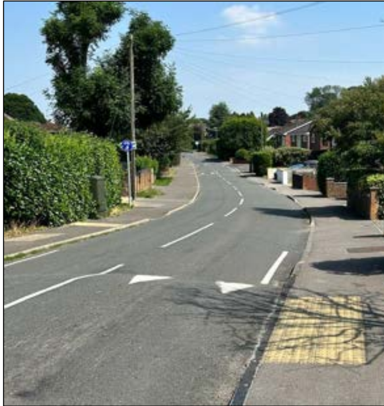
Photograph 87: Raise Table Tactile Paving Crossing on Victory Avenue
