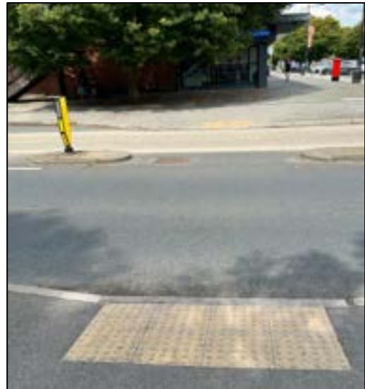
Photograph 50: Crossing Point on Eagle Avenue north of Milton Road Mini Roundabout
