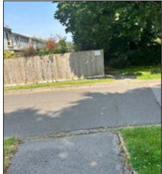
Photograph 55: Footways crossing Spencer Gardens
