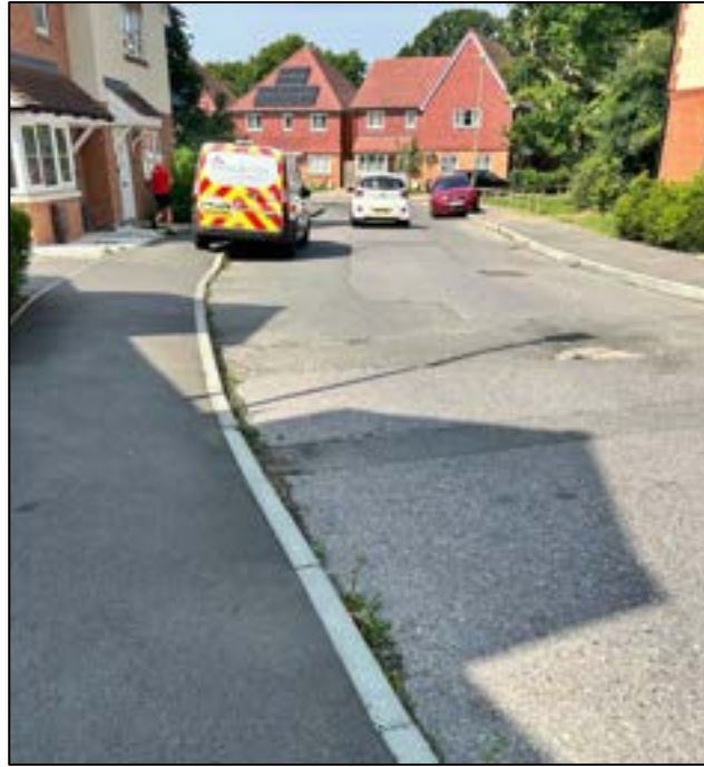
Photograph 17: Footways along Merritt Way west of the Junction of Powell Drive
