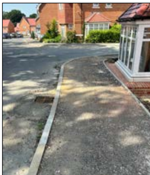
Photograph 23: Existing Conditions along Hudson Gardens
