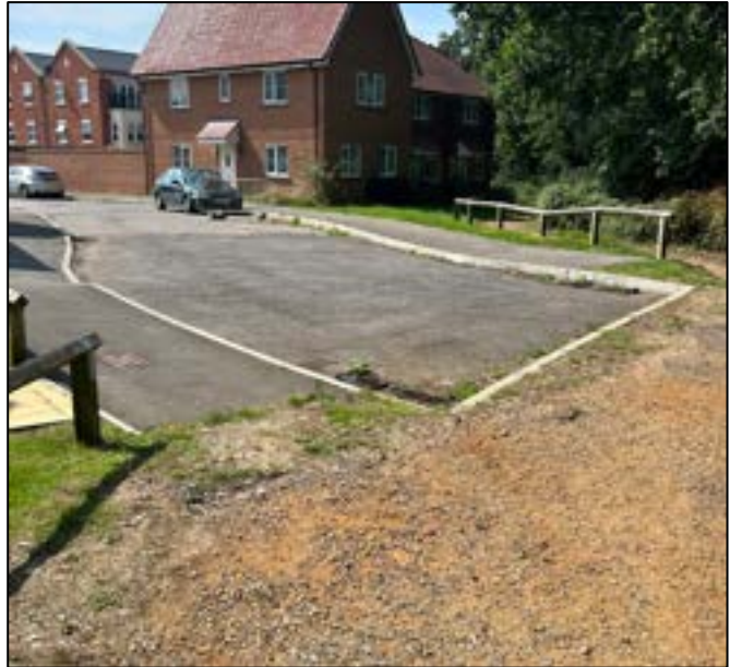
Photograph 15: Existing Dead End and Connection to Bridleway
