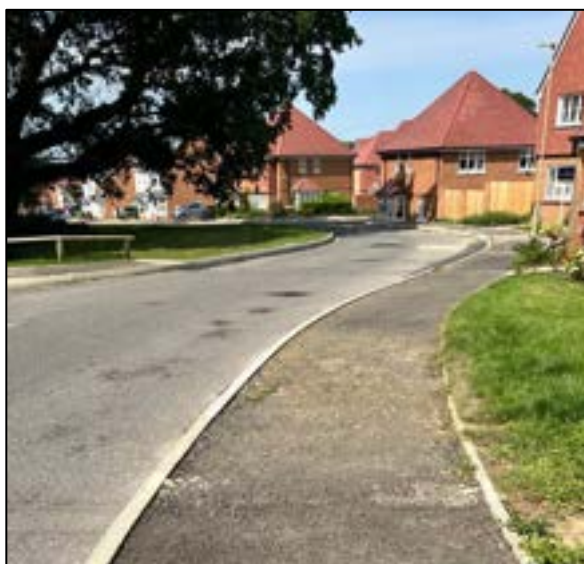
Photograph 22: Existing Conditions along Hudson Gardens
