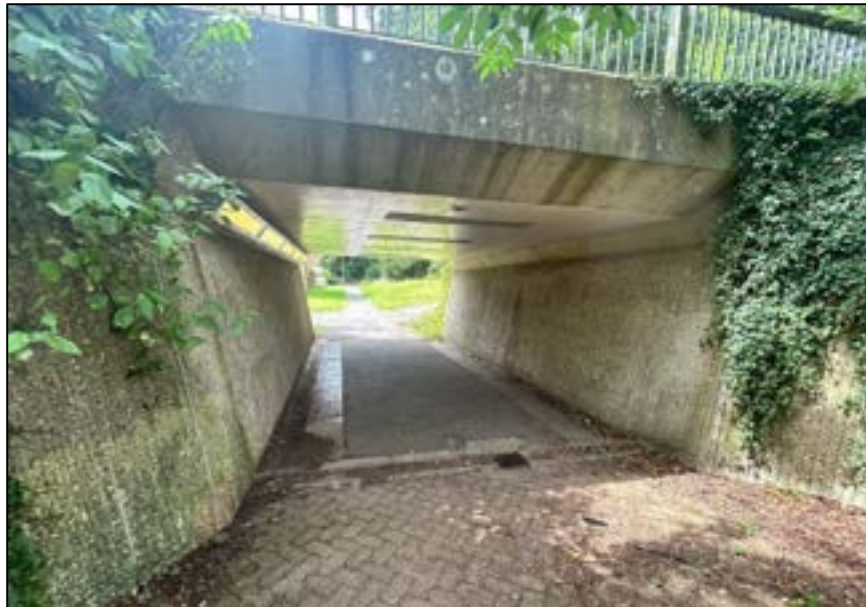
Photograph 59: Underpass between The Acorn Community Centre and the Southern Footways along Eagle Avenue
