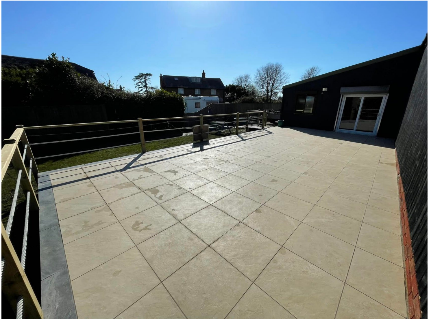
Fig 7. NOTE THAT IMMEDIATELY BEHIND THE TEE CADDY CAFÉ TERRACE CAN BE SEEN ONE OF THE CARAVANS BEING STORED IN THE NON-CONSENTED CARAVAN STORAGE AREA AND THAT THIS LARGE OPEN DINING AREA IS IMMEDIATELY ADJACENT TO 'THE GRANARY', ONE OF THE TWO RESIDENCES THAT A G PHILLIPS & SONS LTD CLAIM TO BE 'LOSING AMENITY' DUE TO THE USE OF TOURNERBURY WEDDING VENUE RIGHT OF WAY.
