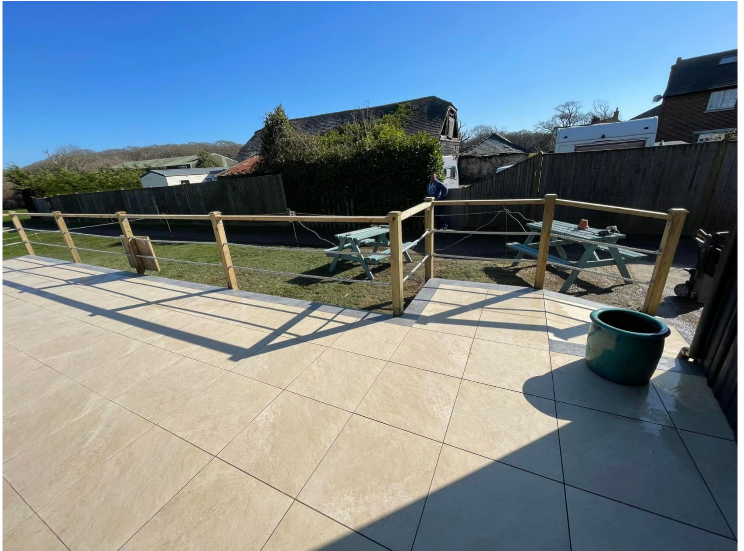
Fig 8. AS ABOVE – NOTE IMMEDIATE PROXIMITY TO ‘THE GRANARY’ DWELLING AND TWO CARAVANS BEING STORED IN THE UNCONSENTED ‘CARAVAN STORAGE AREA’ CAN BE SEEN HERE. TO THE LEFT OF THE PHOTOGRAPH THE NON-PLANNING CONSENTED STATIC CARAVAN THAT IS COMMERCIALY LET BY MR AND MRS PHILLIPS CAN BE SEEN BEHIND THE FENCE.
