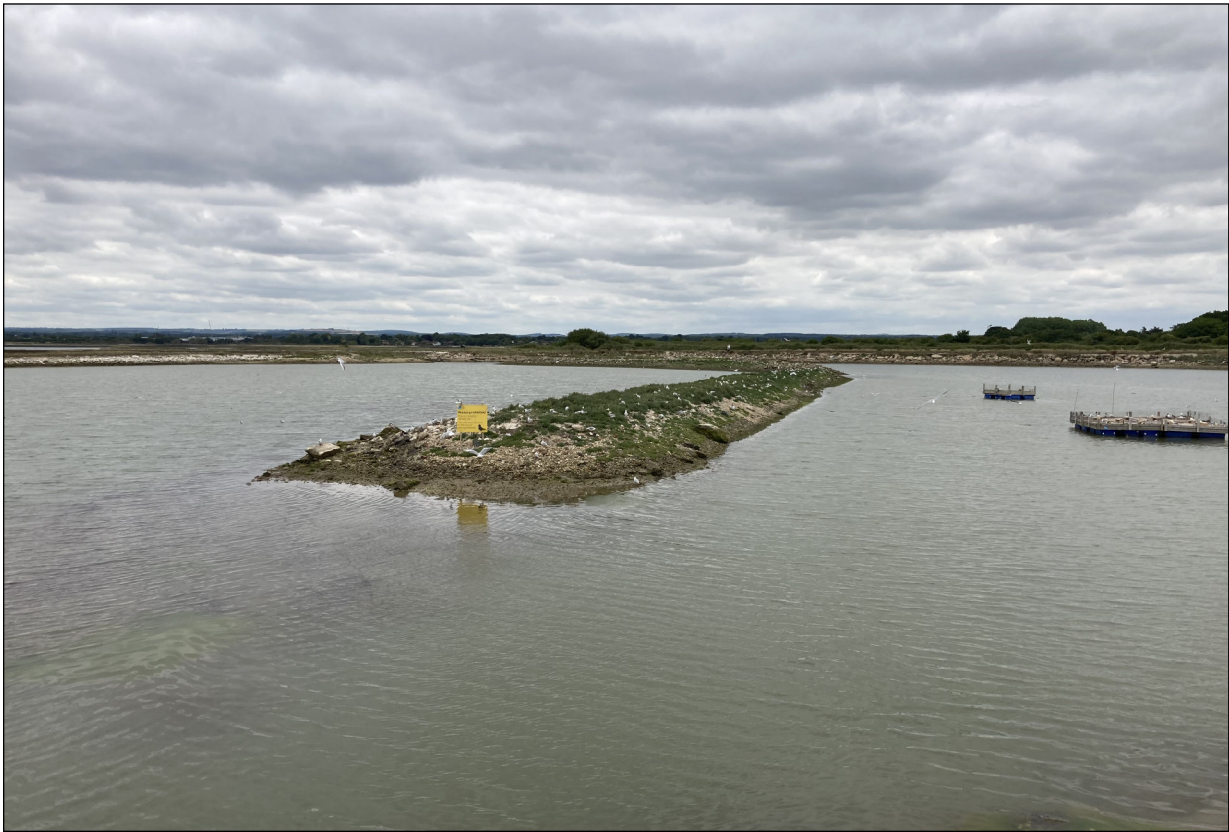
Plate 1) The remains of the bund wall within the lagoon off Creek Point, where shingle will be deposited. Taken facing north.
