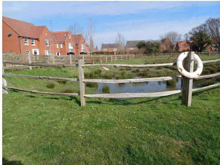
Photograph 1: Northernmost SuDS basin
