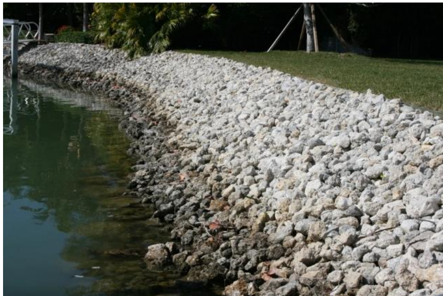
Figure 1 - Example RipRap on an Riverbank [1]
