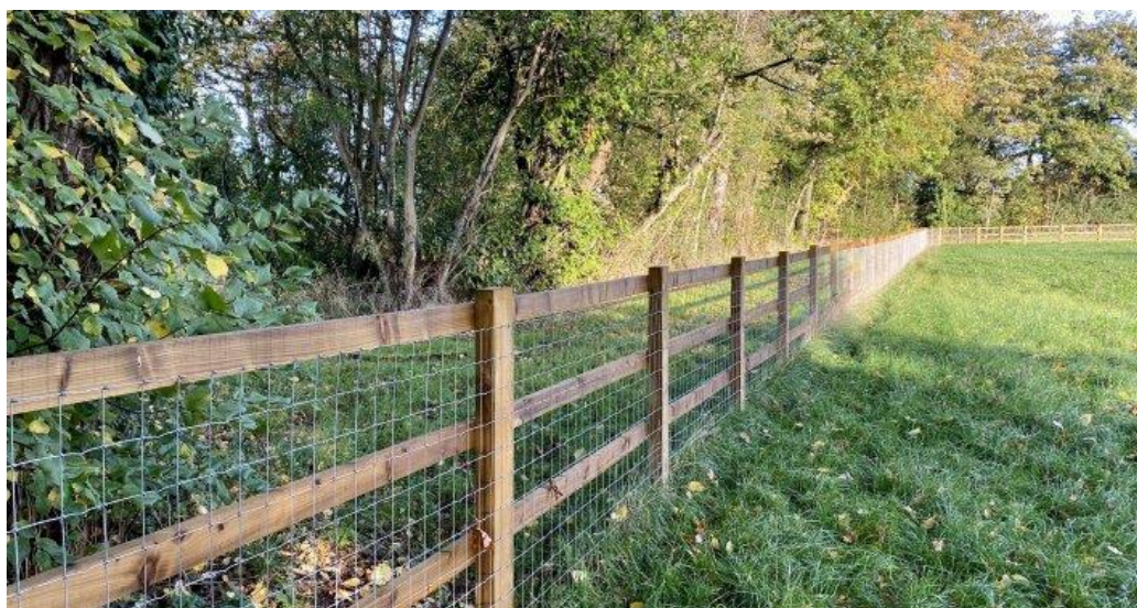
Figure 2 - Typical Livestock Proof Post & Rail Fence [2]
