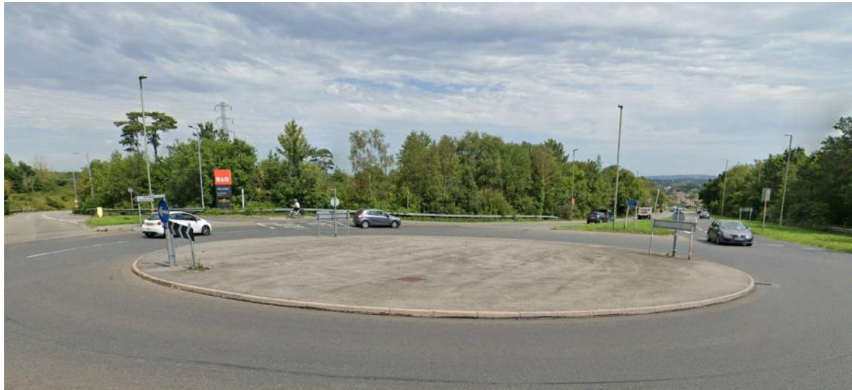
Site approach from the roundabout on Purbrook Way
