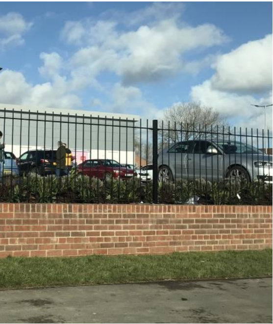
1100mm high railings
