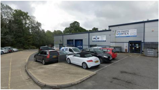
Commercial / Industrial Units
