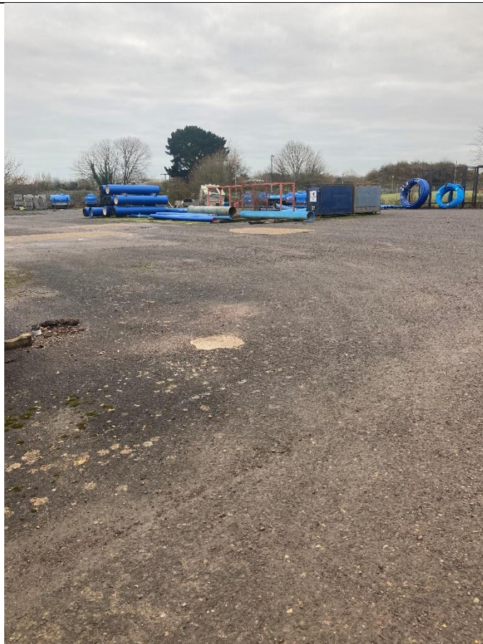
Photograph 1: View of hard standing typical of the site
