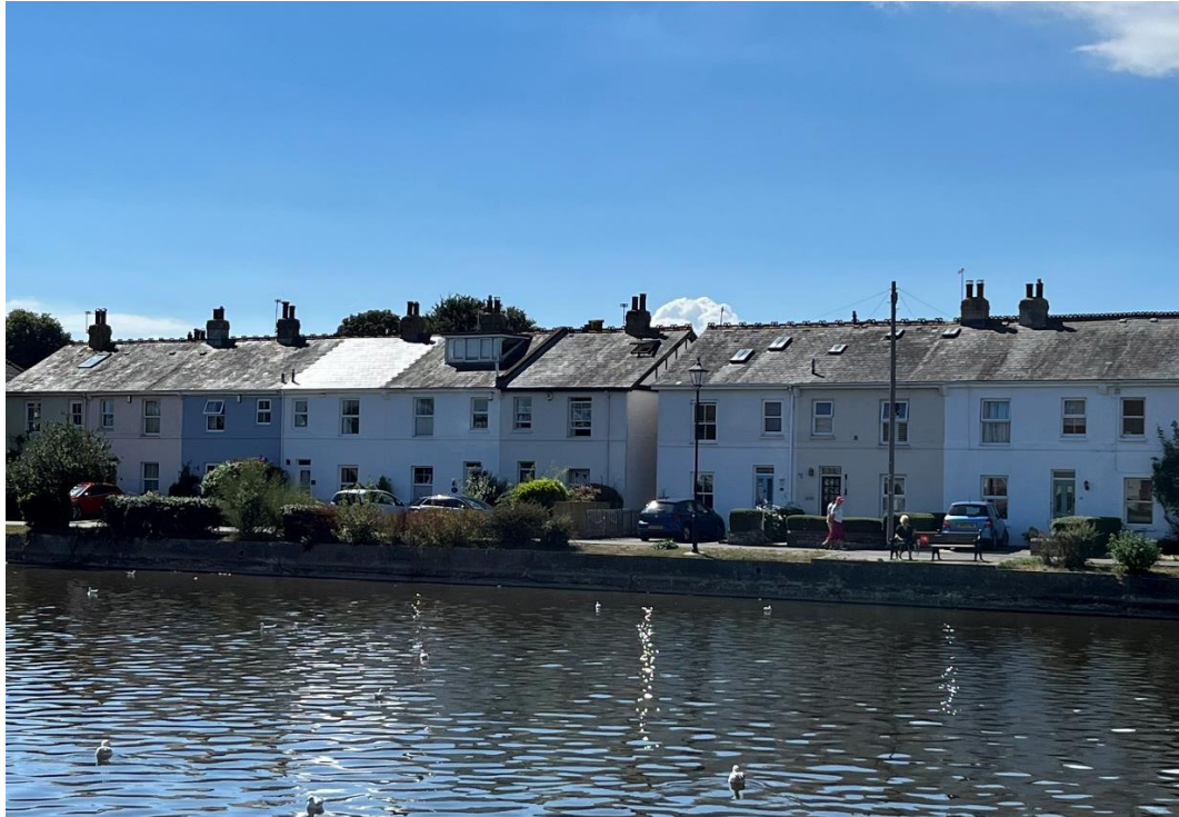
Figure 6: 30 Bath Road in Street Elevation, as seen from top end of Bridgefoot Path.
