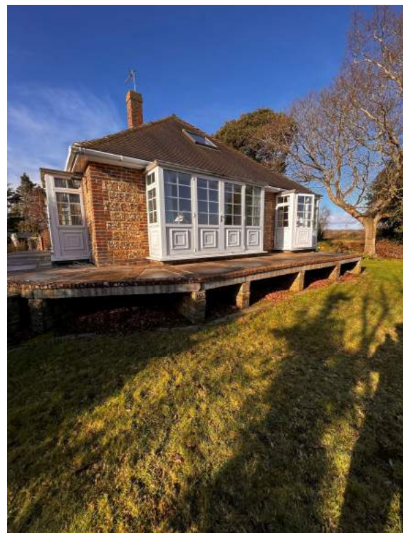
Existing House East
