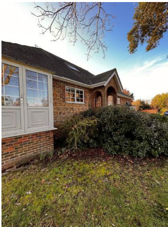
Existing House North
