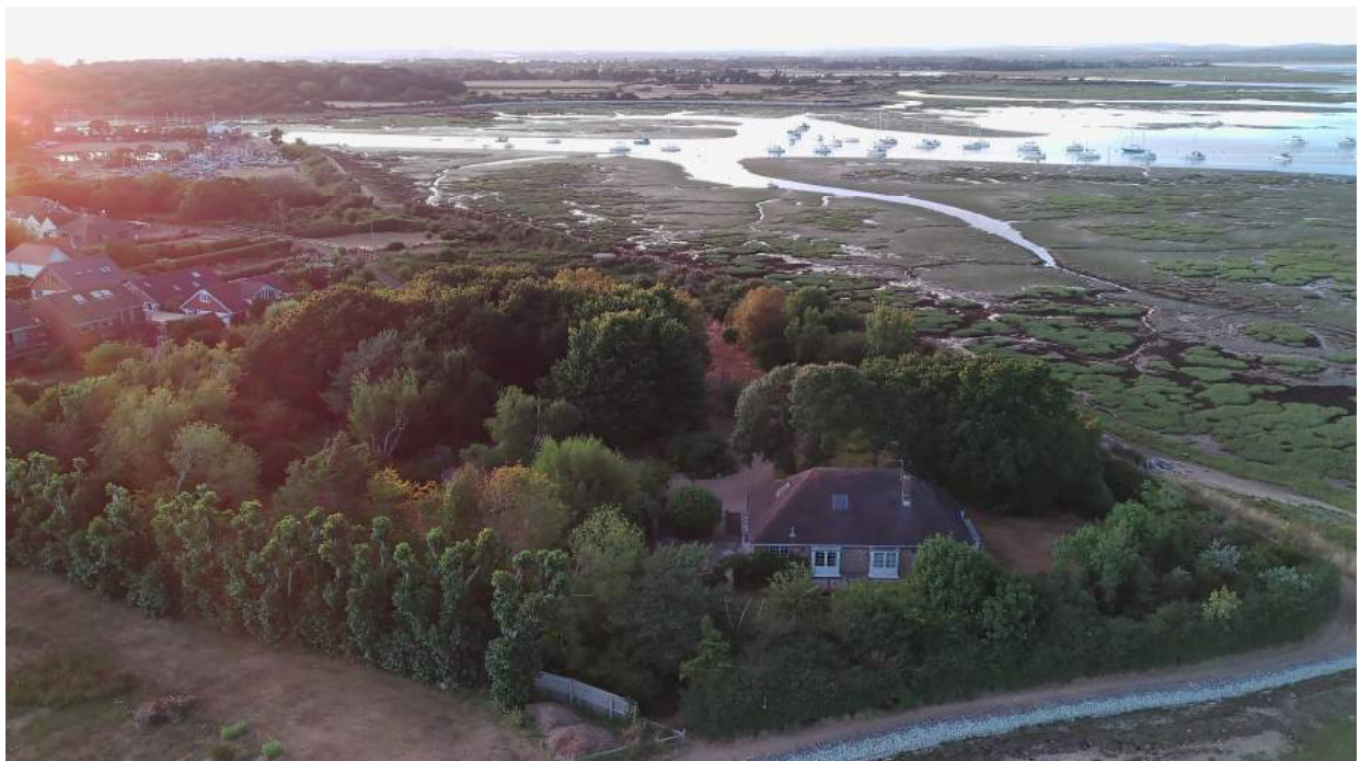
General View to North
