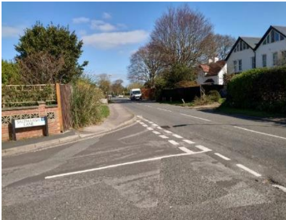
Photograph 5: Dropped kerbs at the junction of Saltmarsh Lane and West Lane.
