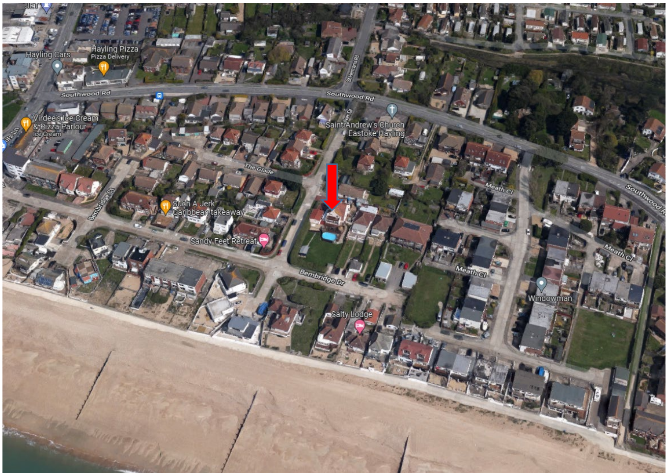
Image 1 – Aerial View of the Site
