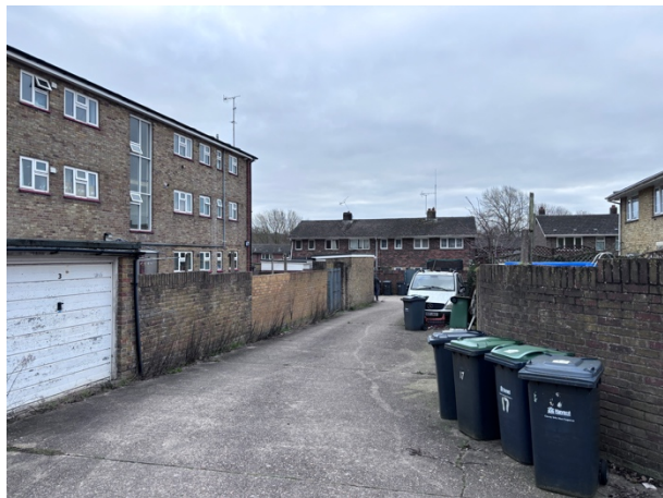
The site viewed from the west on communal access drive.
