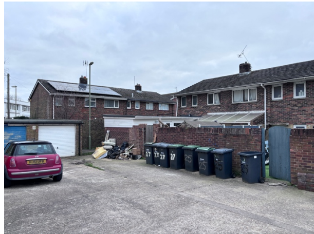
The site viewed from the west, on the communal service area.
