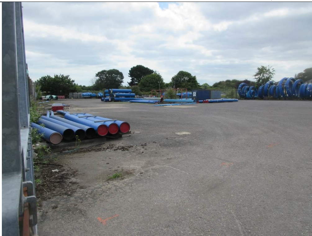
Plate 5: Western part of site, looking south
