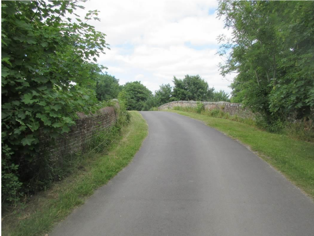
Plate 8: 19 th century bridge over railway, west of site
