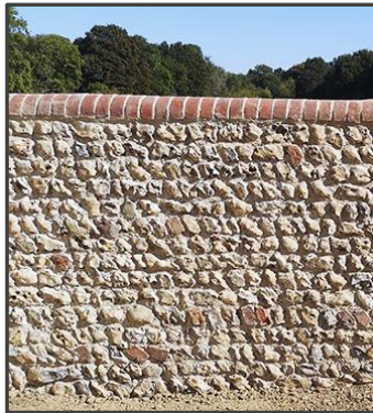
Traditional flint wall with curved brick top detailing.
