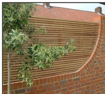
Planting allowed to climb timber fencing.
