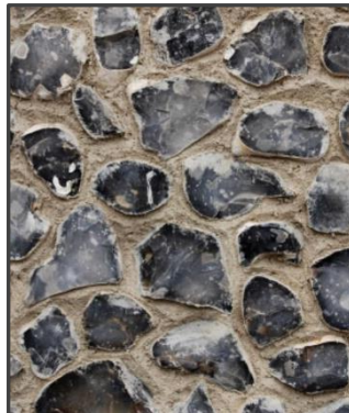
Flint detail with lime mortar
