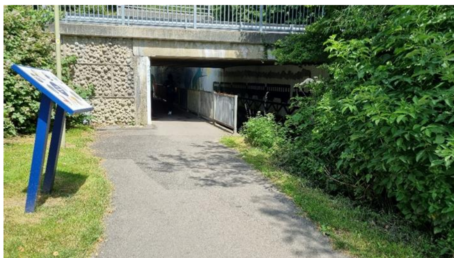
A27 Underpass viewed from south
