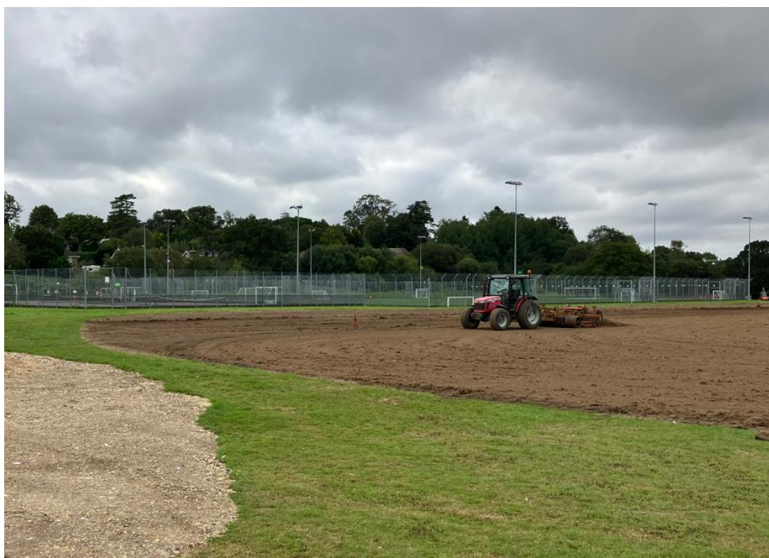
Picture 4: Pitch Construction underway
