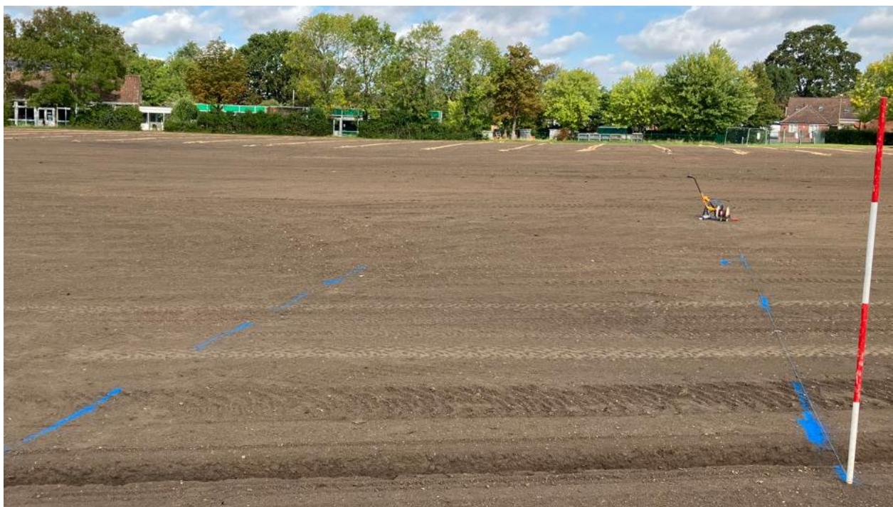
Picture 12: View across new sport pitch with setting out for new lateral drains at 4m c/c
