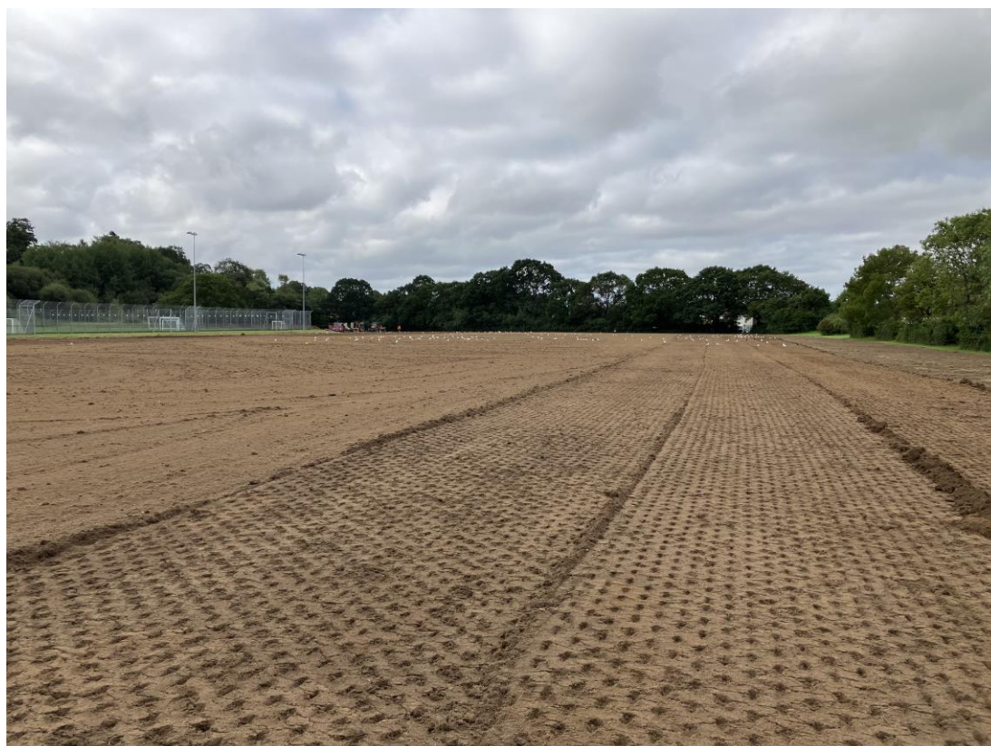
Picture 8: Pitch Construction underway
