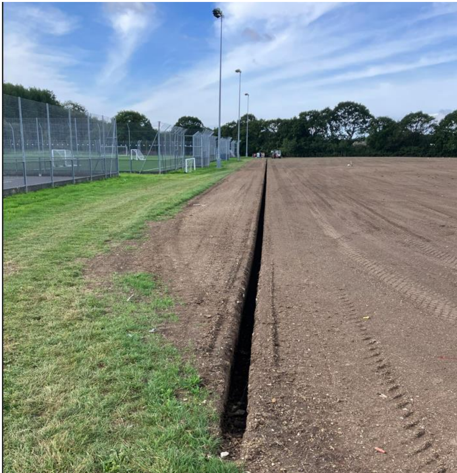
Picture 9: One of the new 100mm dia. Collector Drains
