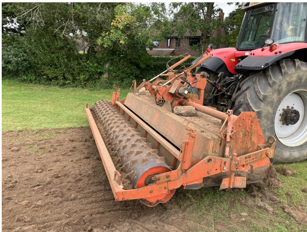
Picture 7: Pitch Construction underway
