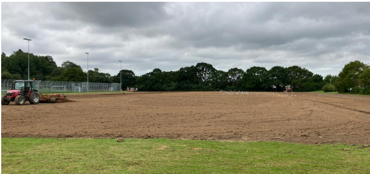
Picture 5: Pitch Construction underway
