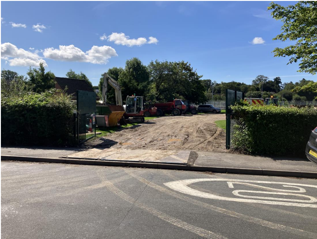
Picture 1: New site entrance with Road/pavement protection plates (kerb plates not yet on site)
