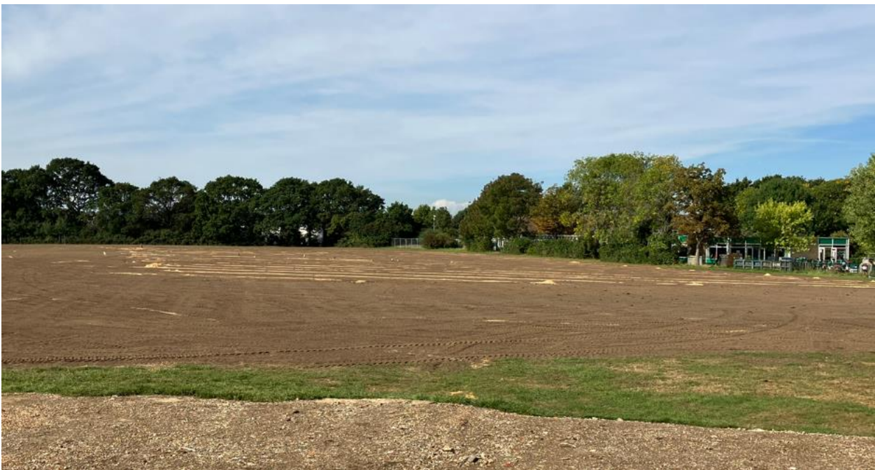
Picture 10: New Sport Sand groves drainage lines
