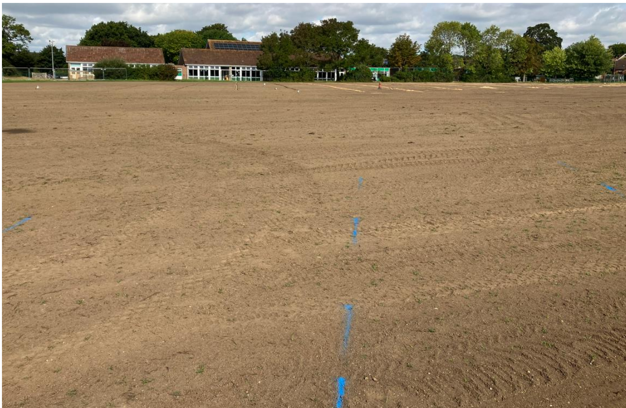
Picture 11: View across new sport pitch with setting out for new lateral drains at 4m c/c
