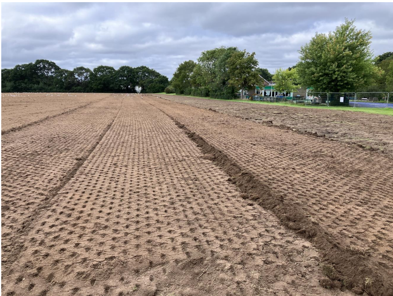
Picture 6: Pitch Construction underway
