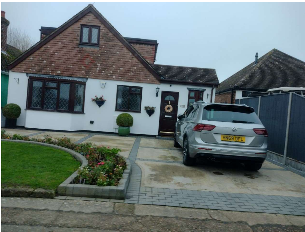
No. 30 Elm Close Estate: Example of side facing dormers and side extension roof
