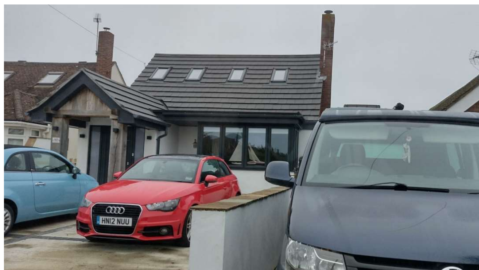
No. 40 Elm Close Estate: Rear Roof Extension and street extension with rooflights
