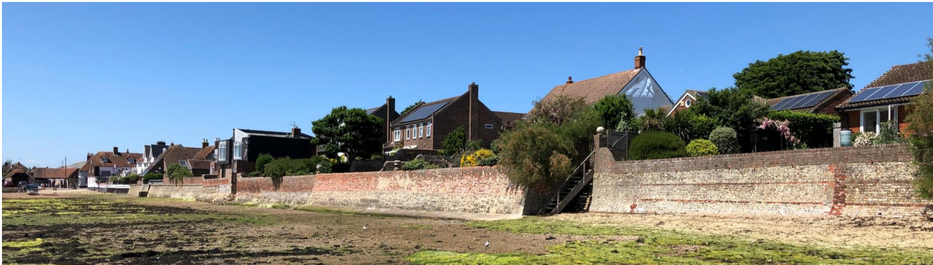
Figure 10 – View of Emsworth waterfront with various brick walls built up off the existing retaining sea wall
