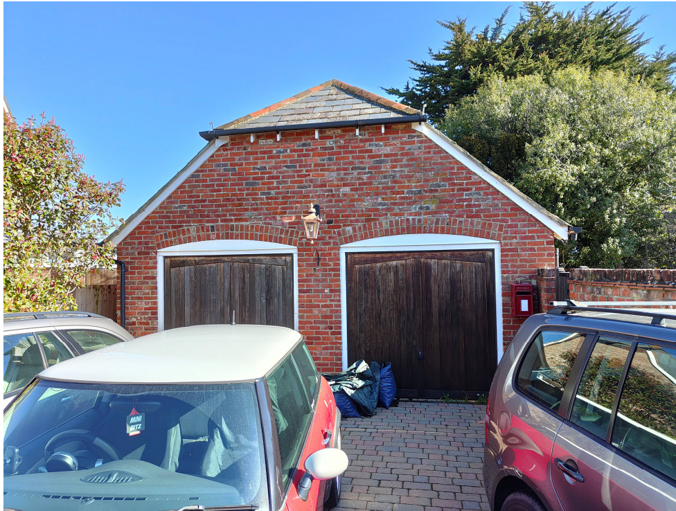
Photograph 1 – showing front elevation of garage / outbuilding
