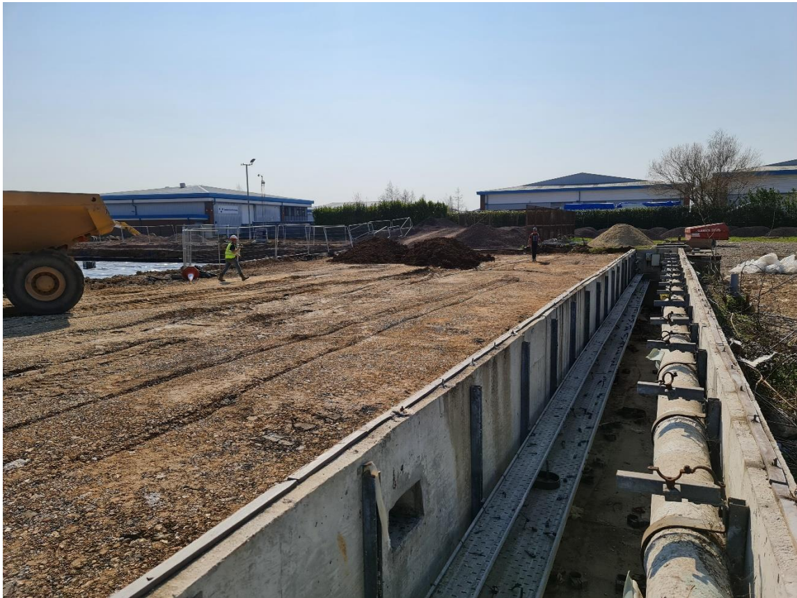
Figure 12 – Stockpiling (suitable) made ground to raise levels to formation
