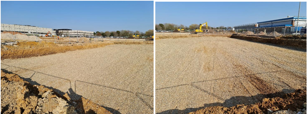
Figure 9 – Attenuation tanks (resulting in mostly natural soils)
