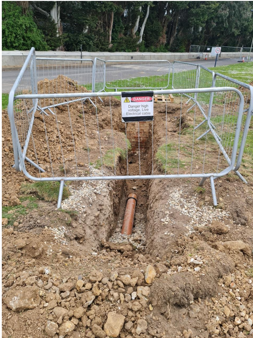
Figure 19 – Drainage work in and around WS2
