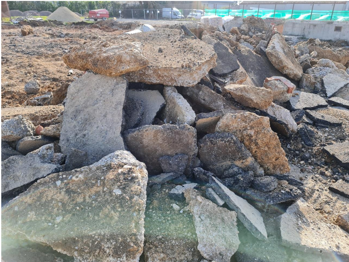
Figure 10 – Oversize and concrete for crushing (NE)
