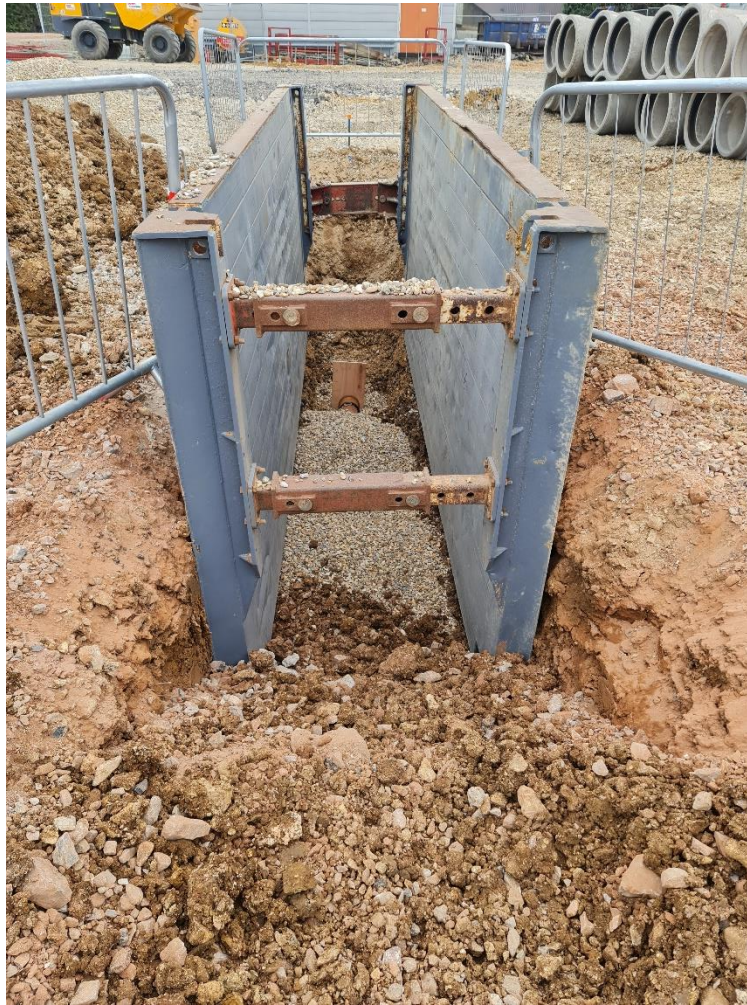
Figure 14 – Ongoing drainage works
