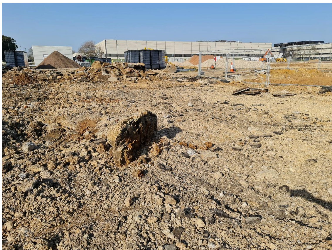
Figure 7 – Southwest development platform - Hardstanding and topsoil removed
