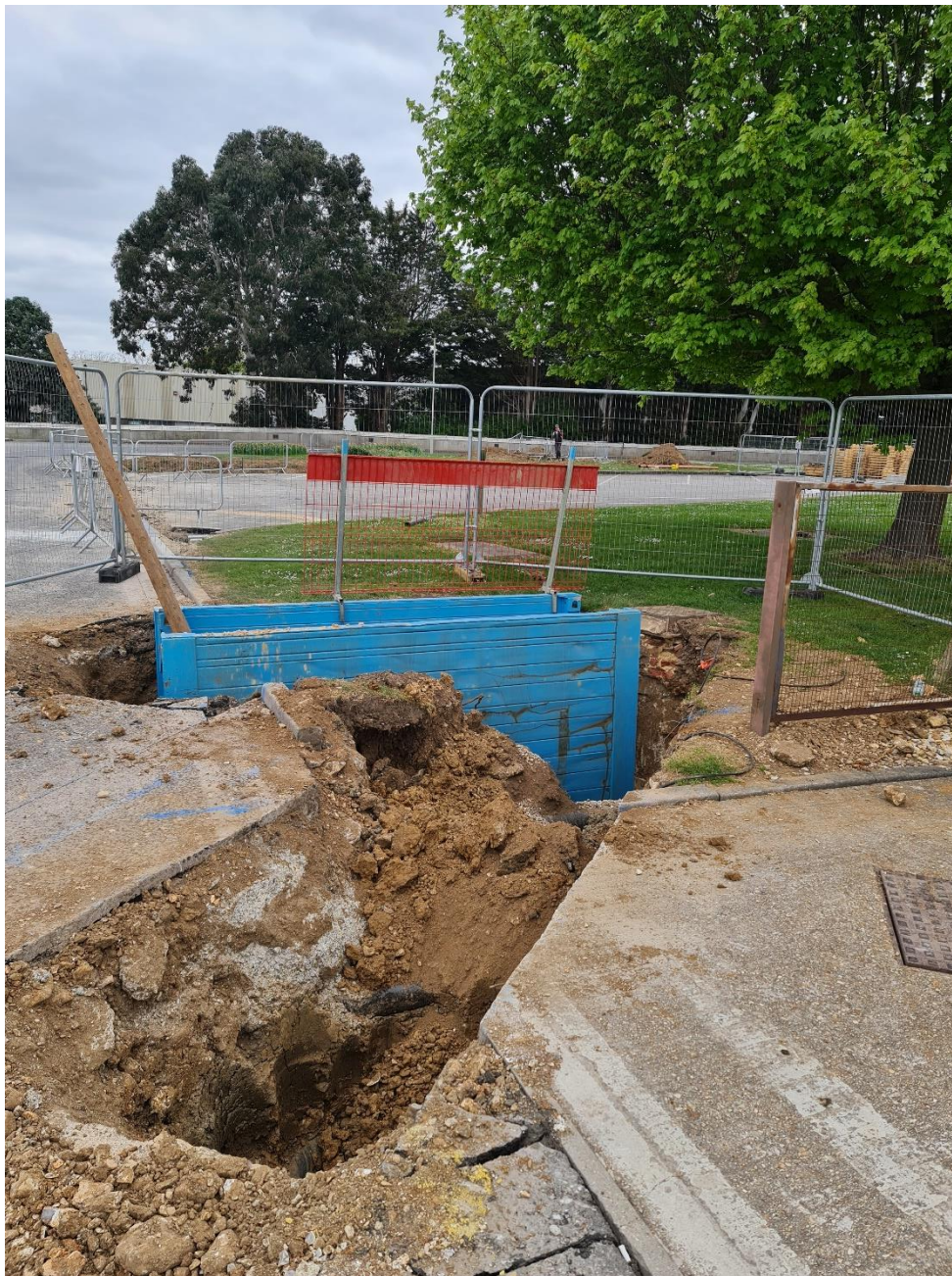
Figure 16 – Drainage work in and around WS2
