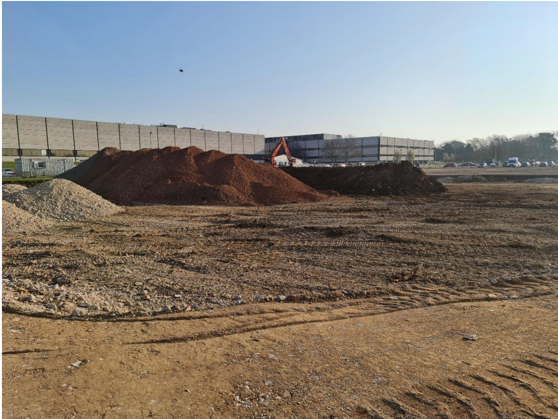
Figure 11 – Use of made ground and imported aggregate to create formation levels and subbase for building slab
