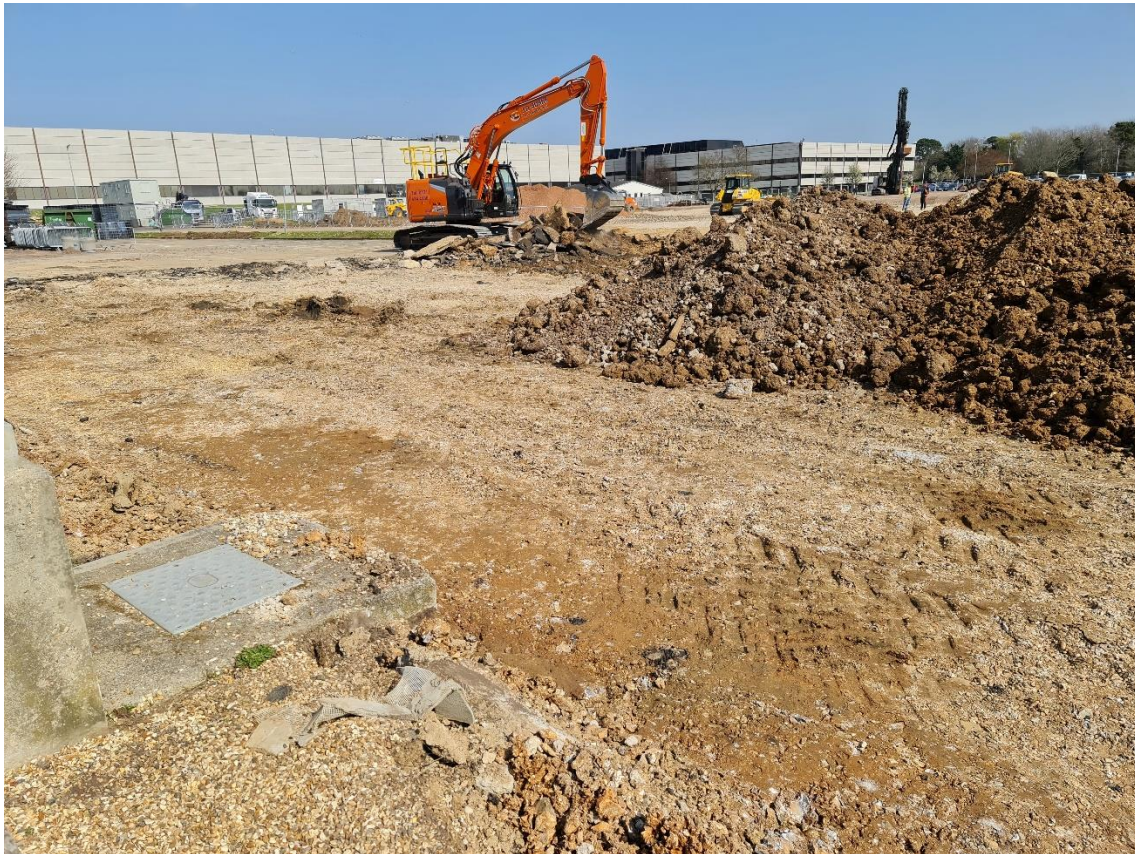
Figure 8 – Segregation of soils (made ground to be reused in SW and concrete for crushing in NE)
