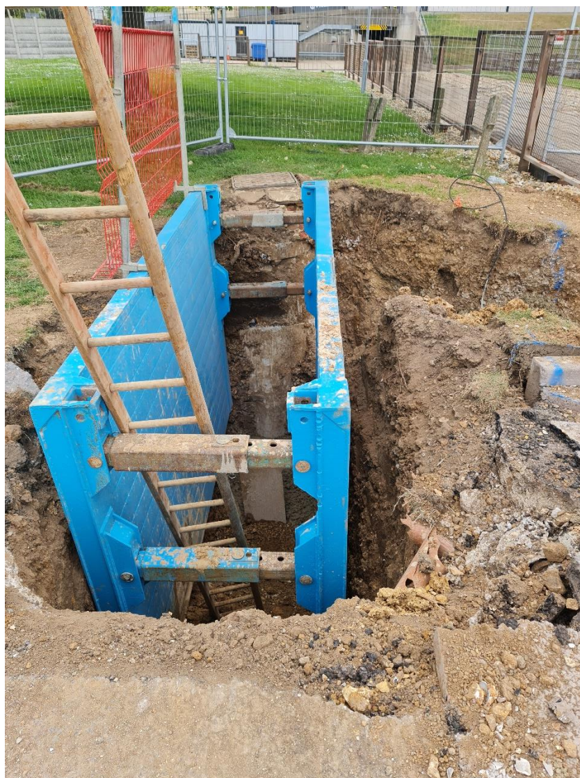
Figure 15 – Drainage work in and around WS2
