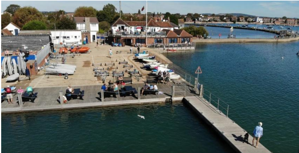
Emsworth Sailing Club – View from South. Sail Shed seen to left (timber building).
