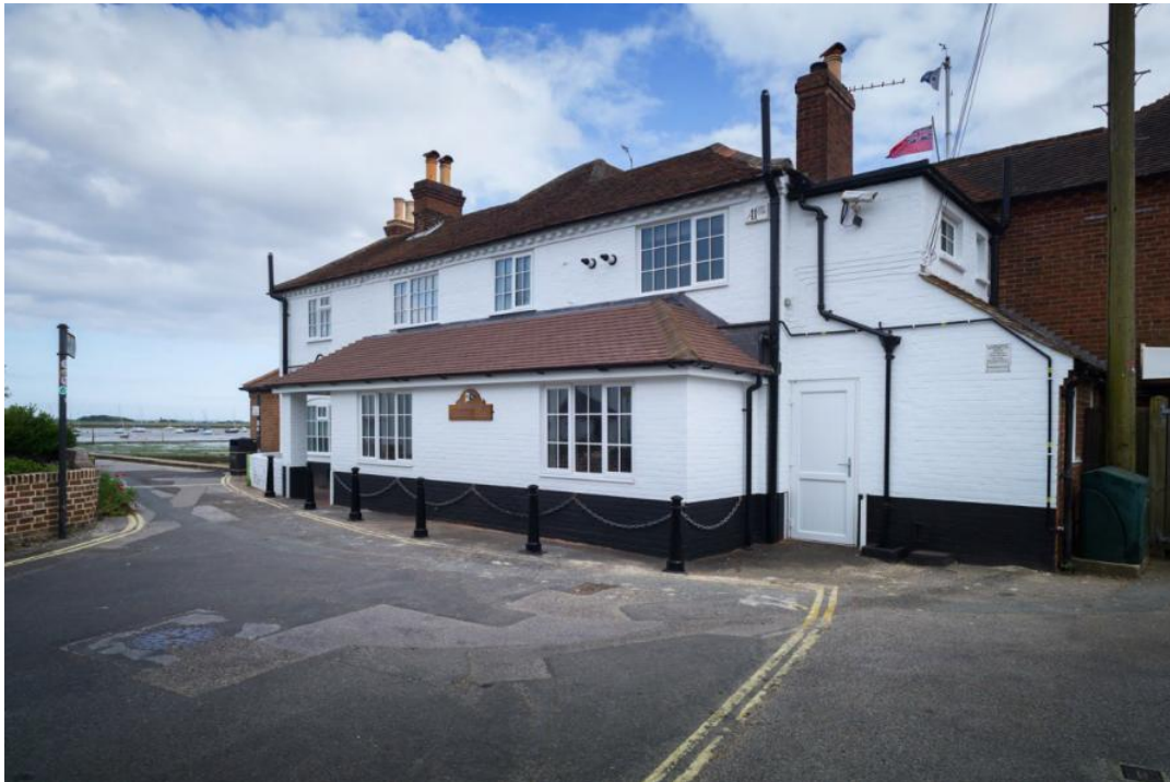
Emsworth Sailing Club – View from Bath Road
