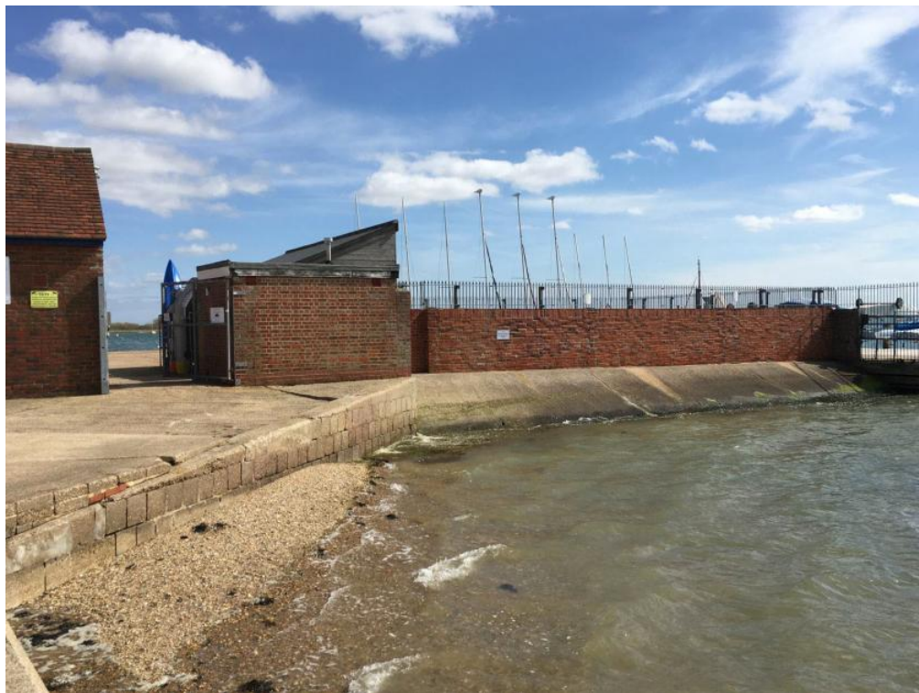
Emsworth Sailing Club – View from West. Sloped roof of sail shed seen just beyond brick wall.
