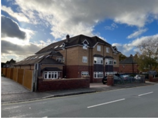
The side (southeast) elevation of the subject building.
