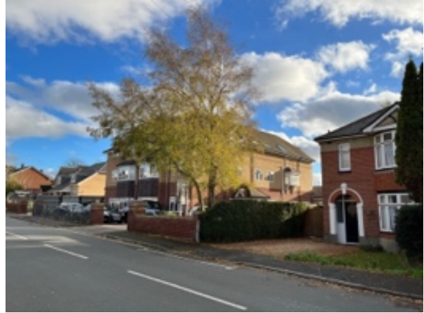
The side (northwest) elevation of the subject building.
