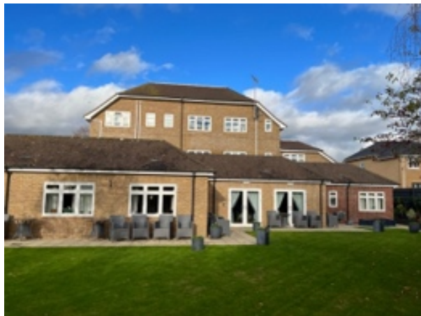
The rear (southwest) elevation of the subject building.
