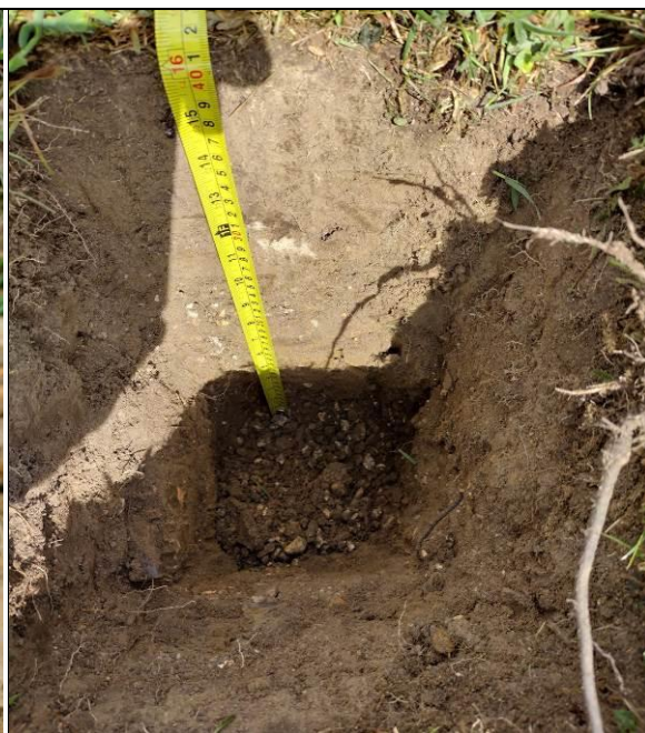
Figure 5. An example of an existing lateral drain. Note the soil contaminated gravel over the drain pipe
