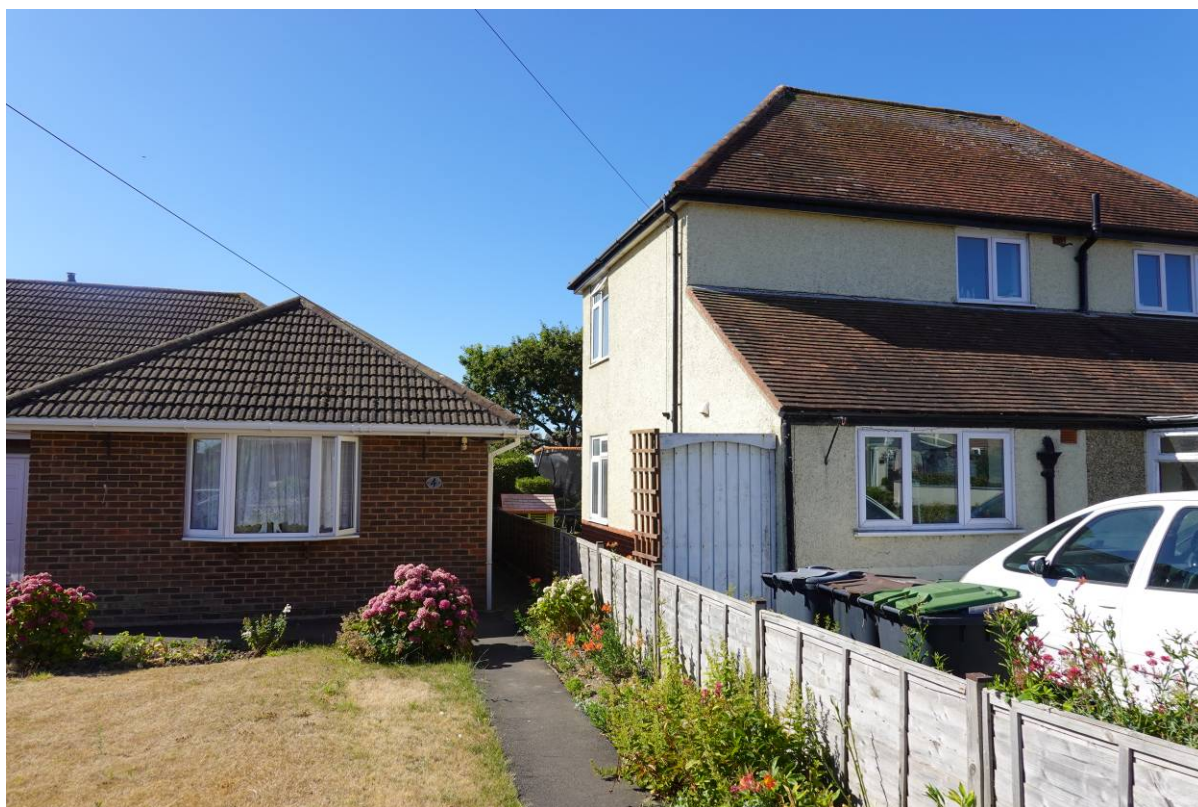
Photo 3 – View of side elevation (east) and No.4 Saint Hermans Road.
