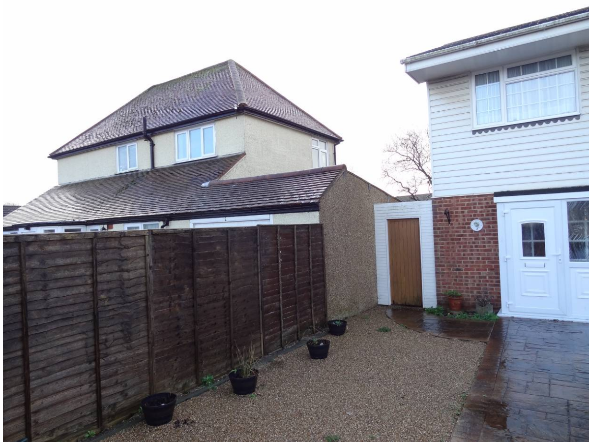
Photo 4 – View of side elevation (west) and No. 2A Saint Hermans Road.
