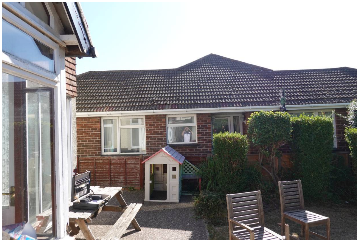
Photo 7 – View of towards side elevation of No. 4 Saint Hermans Road.
