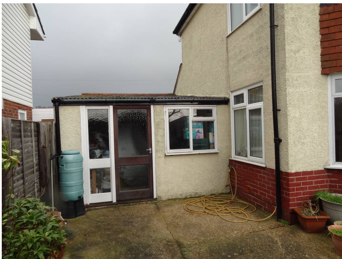
Photo 6 – View of rear of garage to be demolished.
