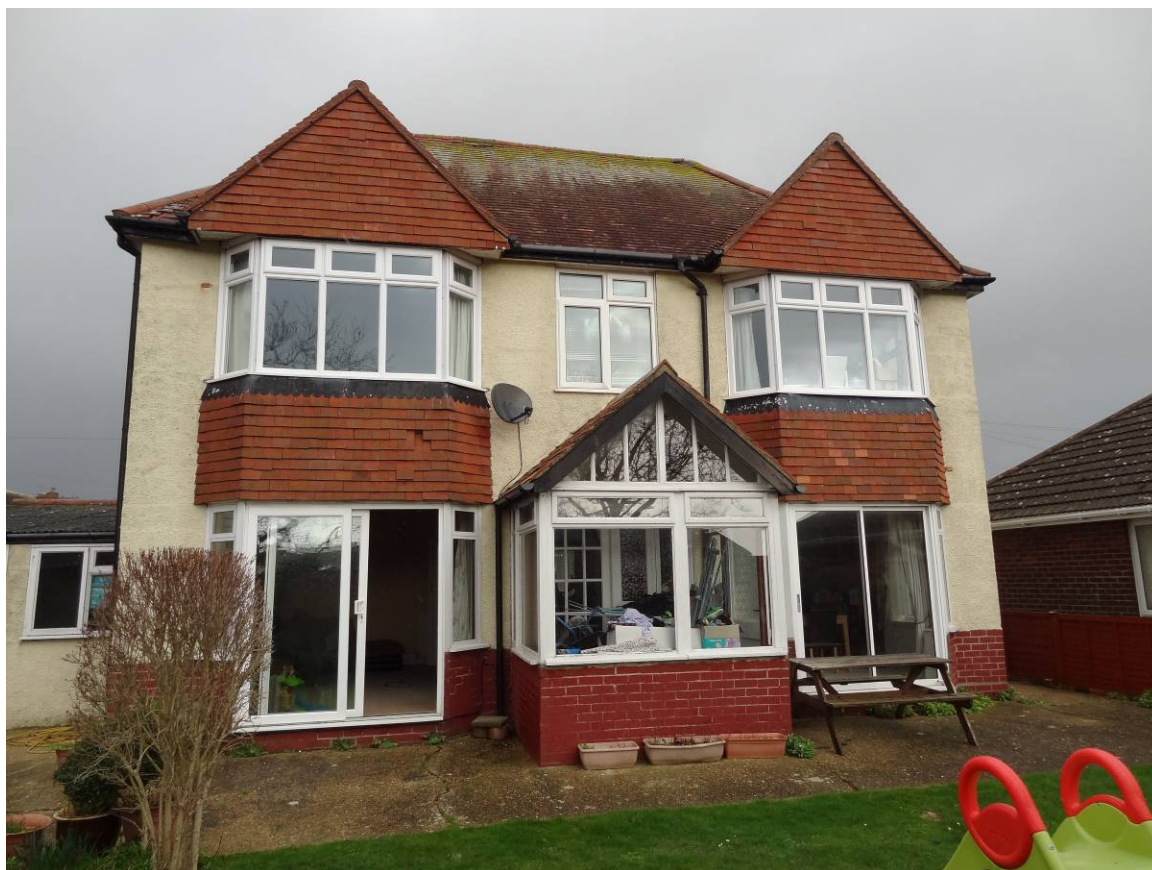
Photo 5 – View of rear elevation (south).
