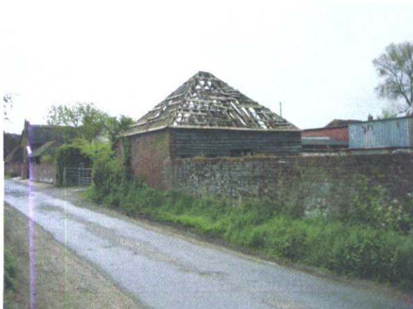
North elevation showing view from Northwood Lane
